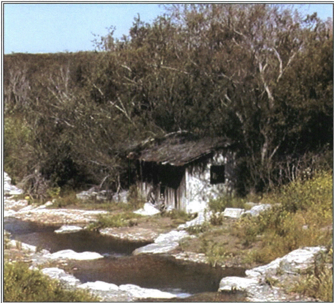
Figure 7.1-1. Historic pump house built in the 1940s, located on Coon Creek within the NRSA.
