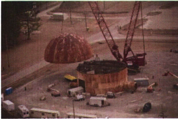
Dome removed from the Hector reactor
