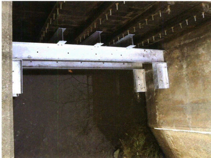
Weir that controls the water level in the canal and the amount of flow in the outlet channel.
