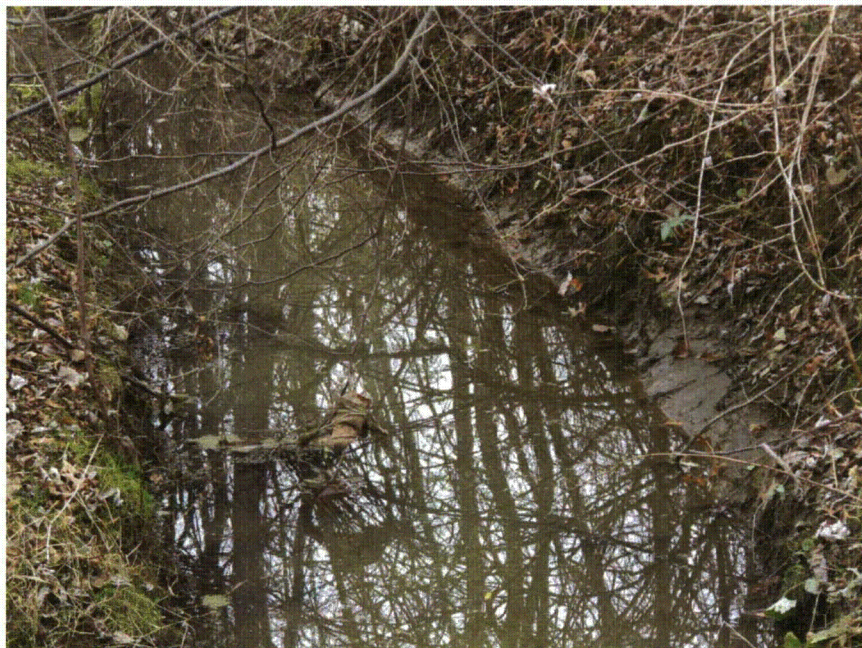
Silt causes turbid water in the upstream section of the outlet channel.
