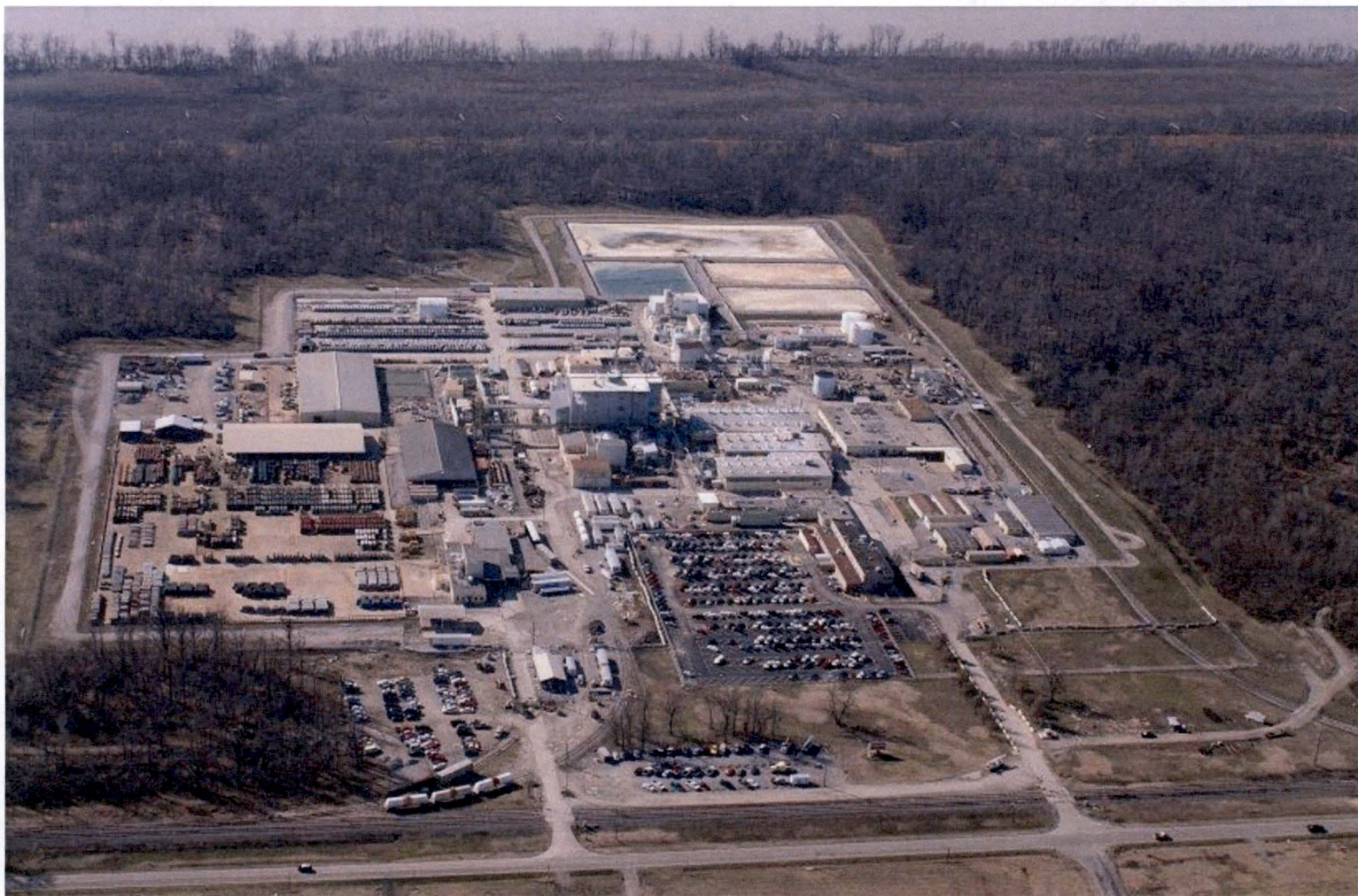
Figure 3.9-1 Aerial View Looking Southwest across U.S. Highway 45 at MTW
