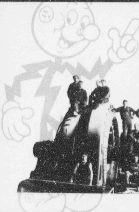
Station 1, an early 100-kV motor generator.
