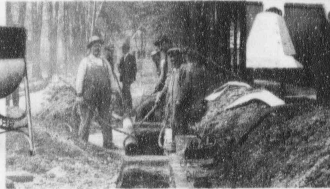
Central heating workers.
