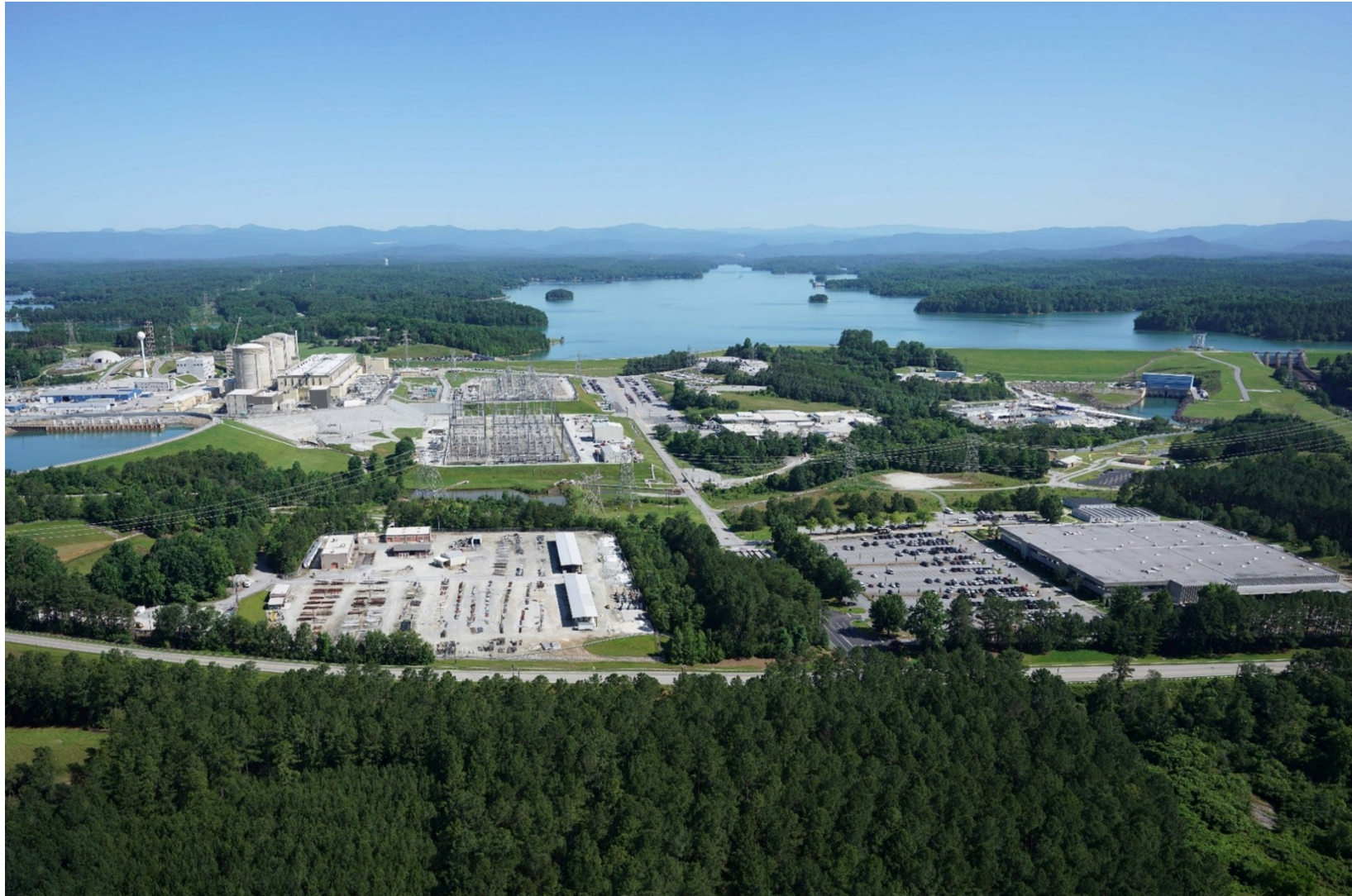
Figure 3.8-8 Post-Construction Photograph of ONS Showing Structures, Buildings, Parking Lots, and Forest
