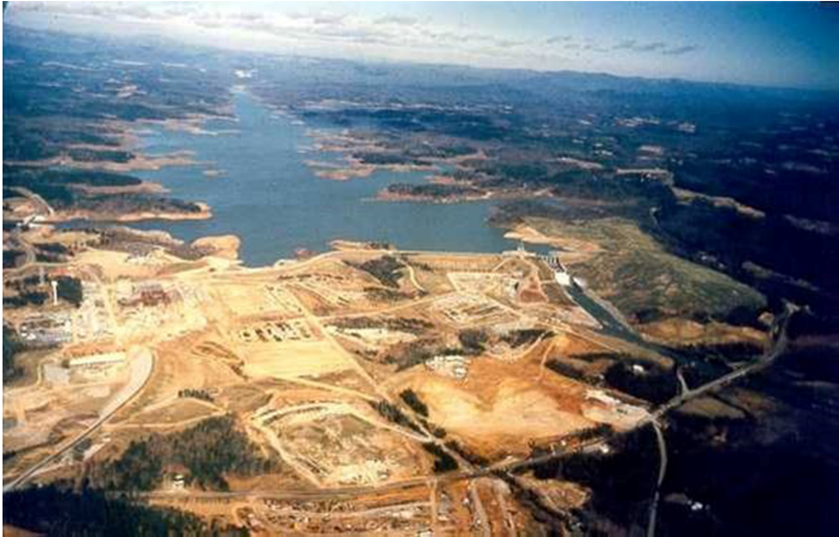
Figure 3.8-6 Construction Photograph of the ONS Site (January 1970) Showing Tree Removal, Lake Keowee, and Mechanical Leveling
