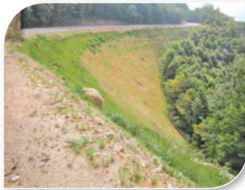
Images from the Foothills Parkway F8E15 project (completed in 2009) show how effective slope stabilization is realized using vegetation. This project is the first project on the east end of the Missing Link Section. The top two images show the slope soon after construction in 2009 and the bottom in 2011.
