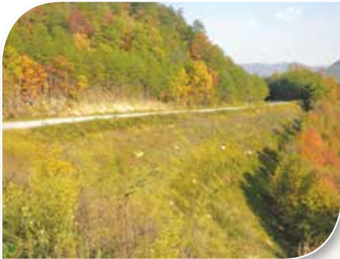
Images from the Foothills Parkway F8E15 project (completed in 2009) show how effective slope stabilization is realized using vegetation. This project is the first project on the east end of the Missing Link Section. The top two images show the slope soon after construction in 2009 and the bottom in 2011.
