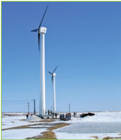
Kasigluk turbines. Ian Baring-Gould/PIX16096.
