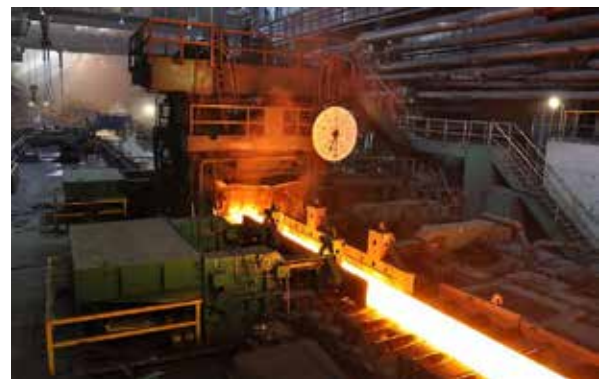
↑ Finishing Section of Hot Strip Mill
