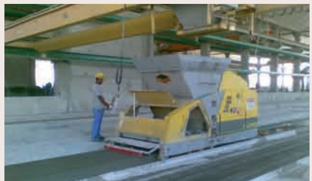
Casting of hollow-core slab
