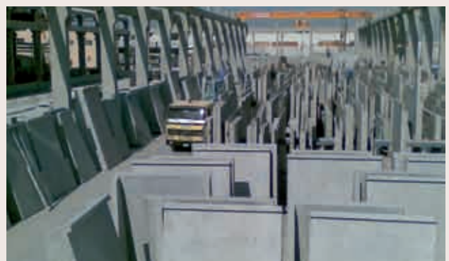
Precast walls in the stockyard
