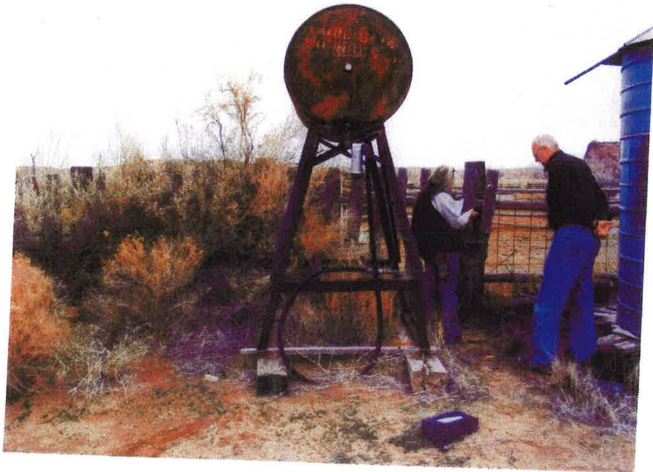
Site 4 – Photograph 19 – Above ground fuel tank appears to be empty, 55 gallon oil barrel, oil spilled on the ground and side of metal granary. Corrals in background.
