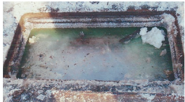
Fig. 1. Handhole prior to deicing.
