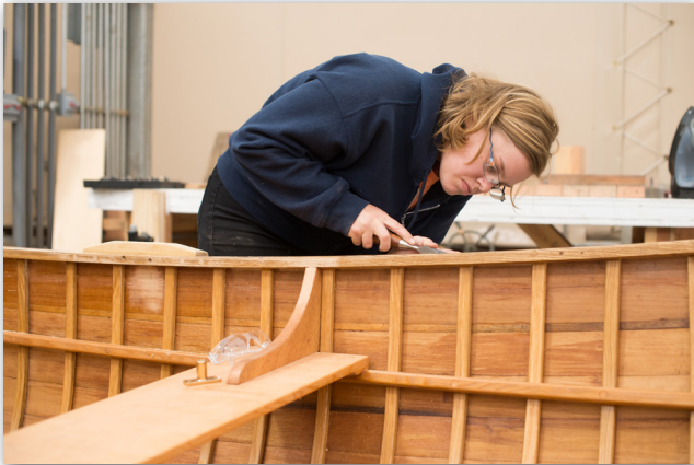
Student Christine aka 'Ducky' uses a chisel for fine details on the Poulsbo boat in the Traditional Wooden Boatbuilding program.
