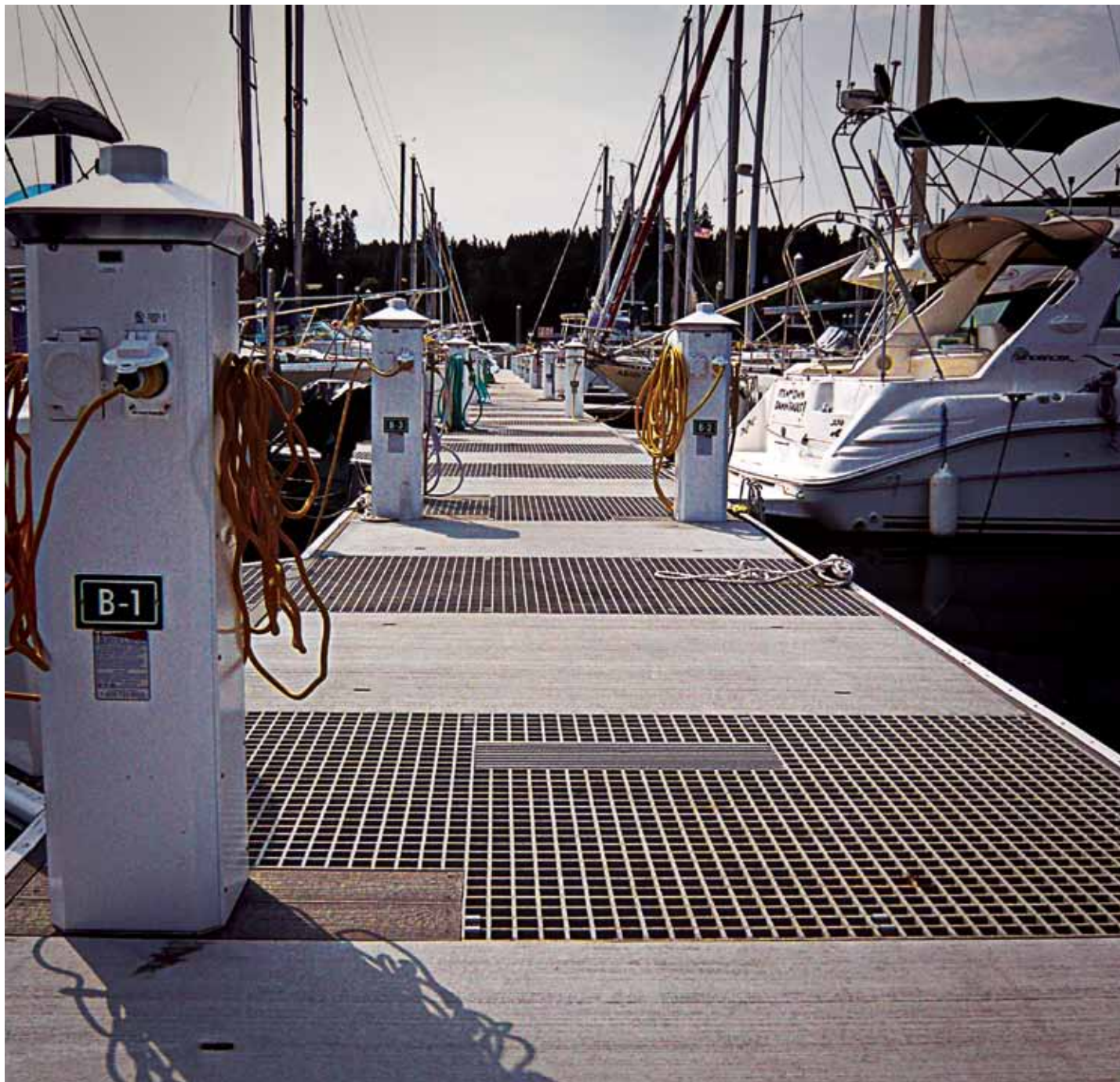
The aerial photo at left was taken after the docks were complete but before docks A and B were refilled with boats. (Dylan Sievert photo). Opposite lower left, the new 80' gangway was one element in bringing Winslow Wharf into ADA compliance. The new docks, complete with grating allowing light penetration (for environmental considerations) were a vast improvement. The Chandlery, which is well stocked, is adjacent to the marina office. Erik Woods photos.
