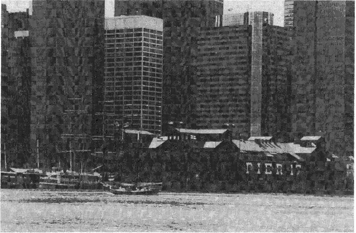
Existing pier redevelopment at South Street Seaport, Manhattan
