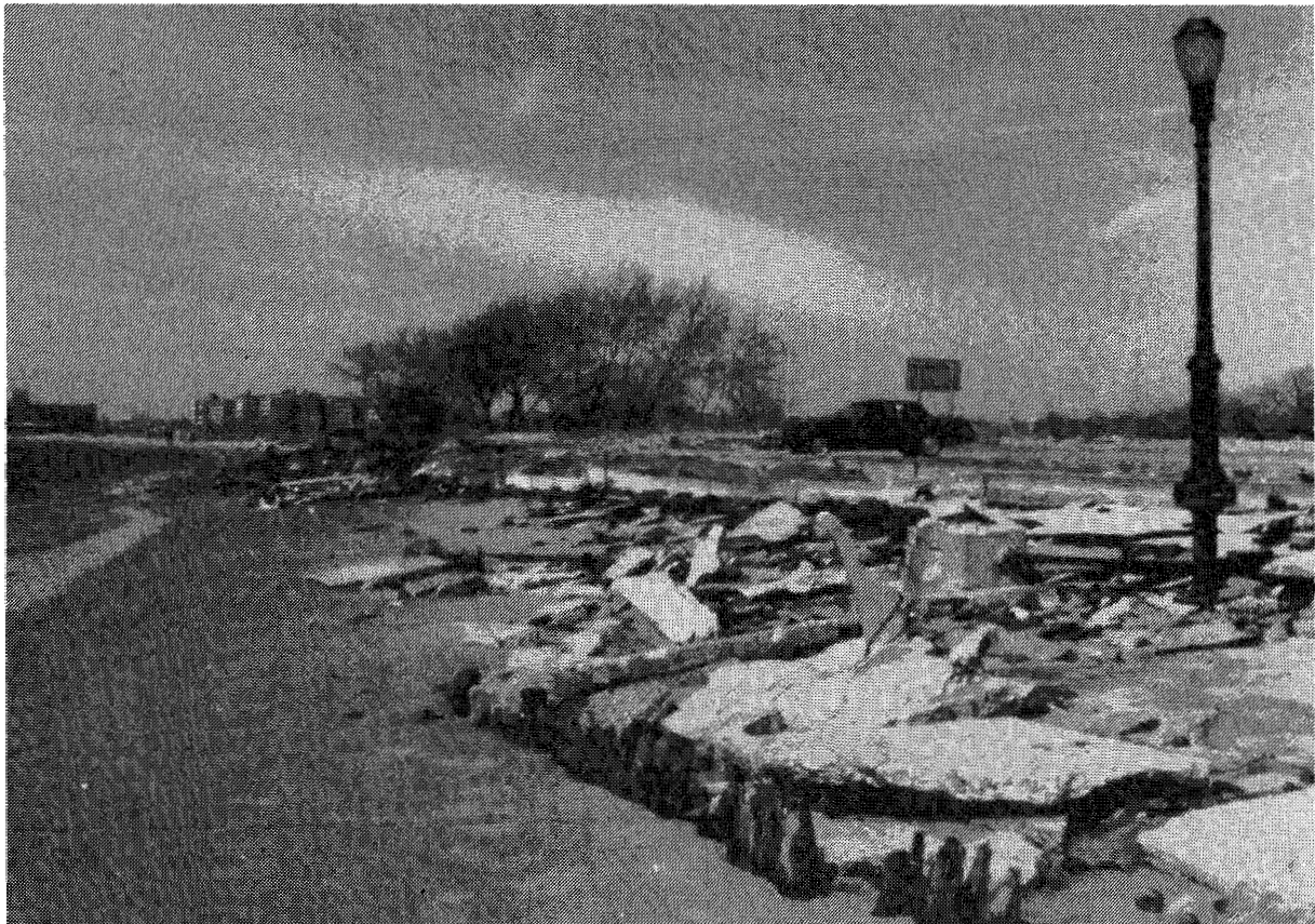
Coastal erosion at Plumb Beach, Brooklyn
