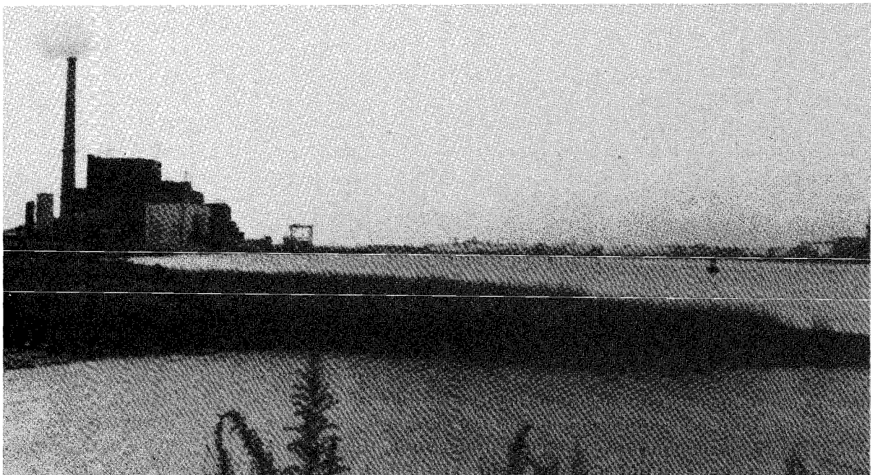
Con Edison power plant on the Arthur Kill, Staten Island
