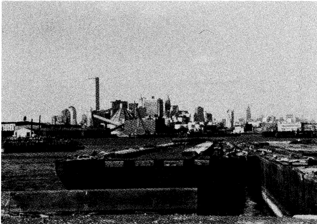
View of Erie Basin from breakwater, Brooklyn
