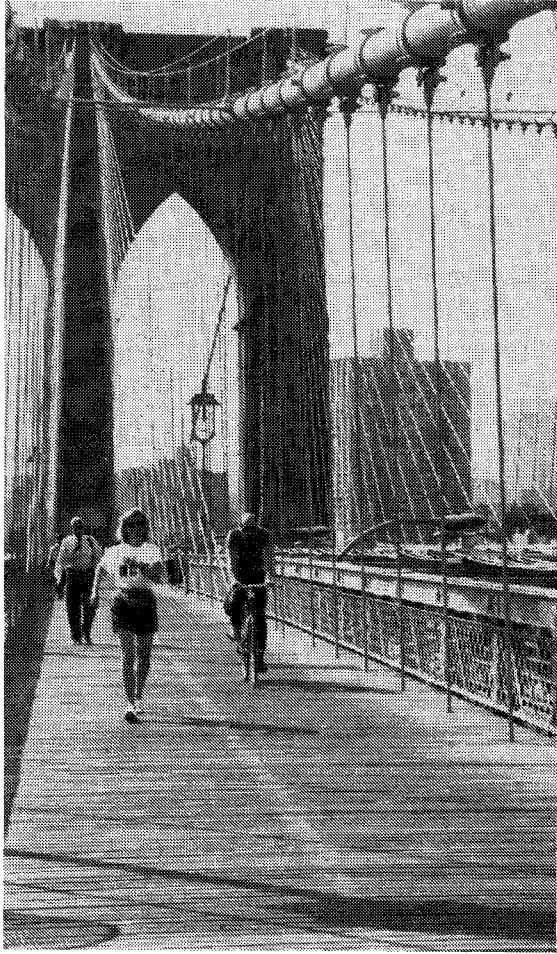
Brooklyn Bridge walkway and bicycle lane
