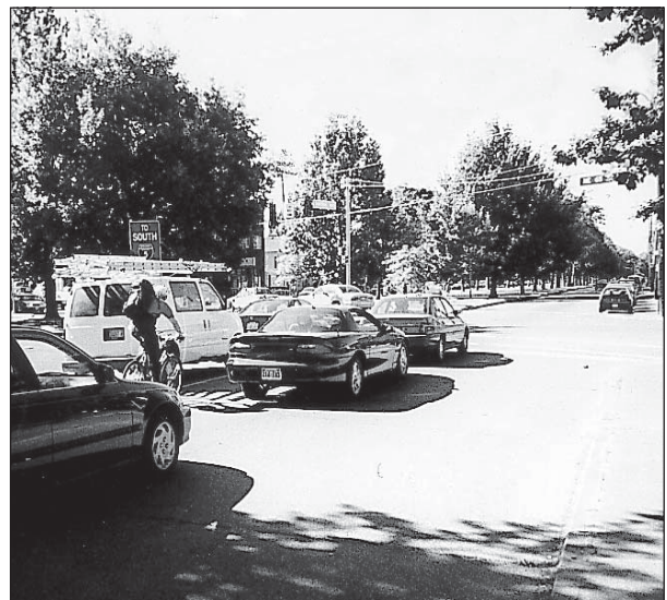
Center-median lane located on Ravenna Blvd. at NE 65th (Seattle) places cyclists between a vehicle left-turn lane and through lane at major intersections.
