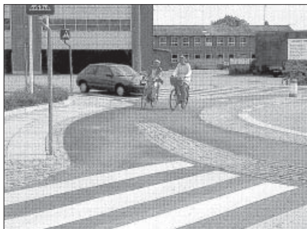
Roundabout with pigmented cycle lanes in Nakskov. Source: Report 106, Road Directorate, Denmark
