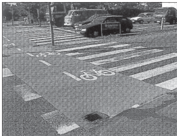
Blue pigmented crossing in Odense (Denmark), used in conjunction with a left-hand broken line marking. Source: Cities Make Room for Cyclists
