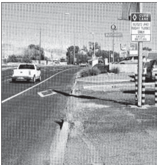
Tanque Verde Rd. bicycle/bus lane (in Tucson).
