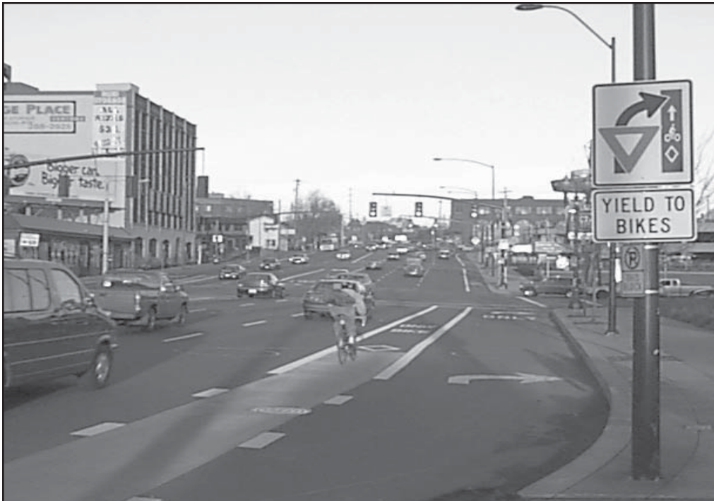
Blue pigmented bicycle lane in Portland, OR, at the east end of the Broadway Bridge. Portland's efforts to reduce conflicts between cyclists and motorists using pigmented lanes are based on research of European techniques. Preliminary evaluation of the lanes has found them to be effective. Source: City of Portland Bicycle web site.
