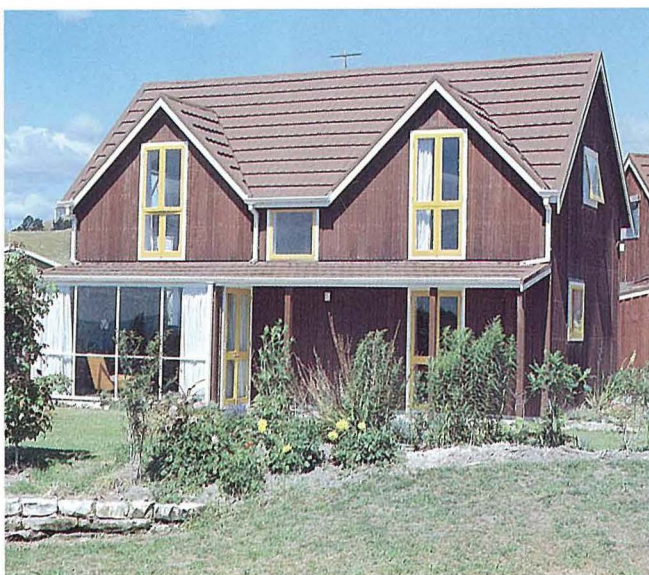
Fig. 14 – New Zealand-grown coast redwood used as exterior cladding on a Rotorua house.
