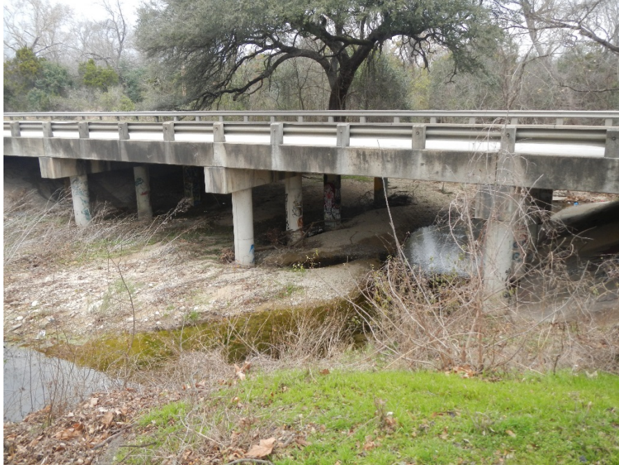
Photograph 17: Williamson Creek at SH 71 bridge; facing northeast.
