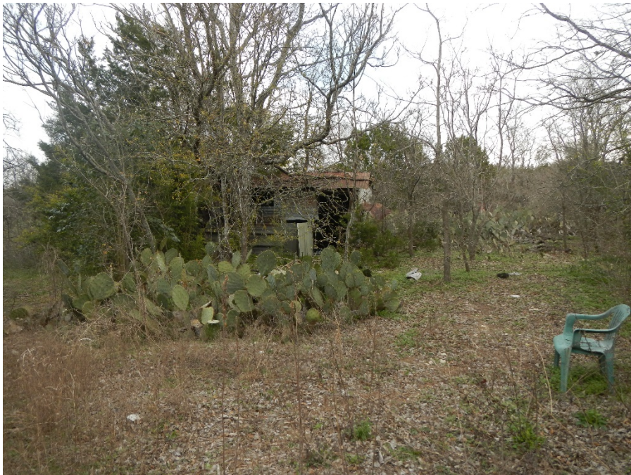
Photograph 36: Debris piles and structure located with the Bee Cave detention pond; facing southeast.
