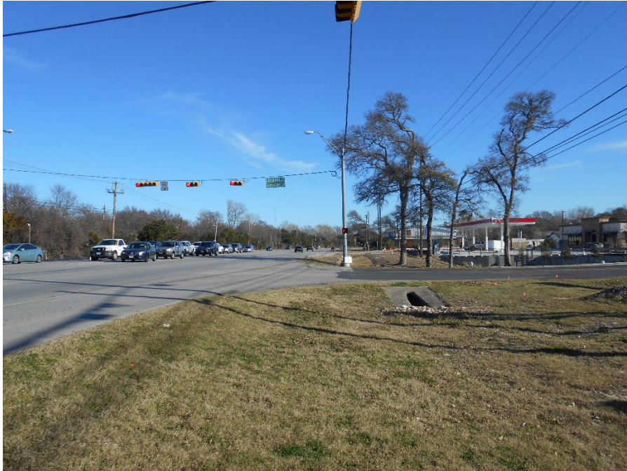
Photograph 29: US 71 at Silvermine Drive; facing south.
