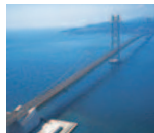
Akashi Kaikyo Bridge (Kobe Side Anchorage)
