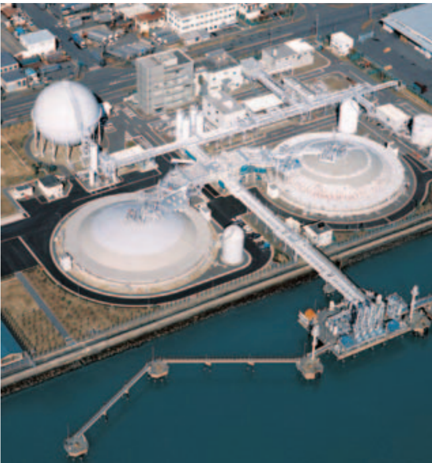
Hiroshima Gas, Hatsukaichi Factory No.2 LNG Storage Tank Location Hiroshima Pref.
