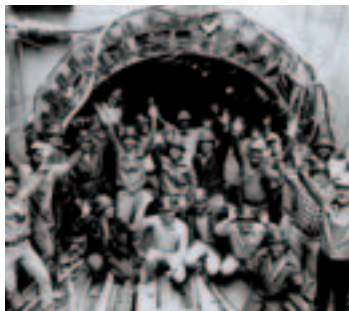
North Shore Outfalls Consolidation Contract N1 & N2
