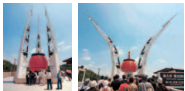
Adaptive Structure by Variable Geometry Truss (VGT) Can be changed into various shapes depending on specific purpose; chosen as a future monument for the Aichi Expo
