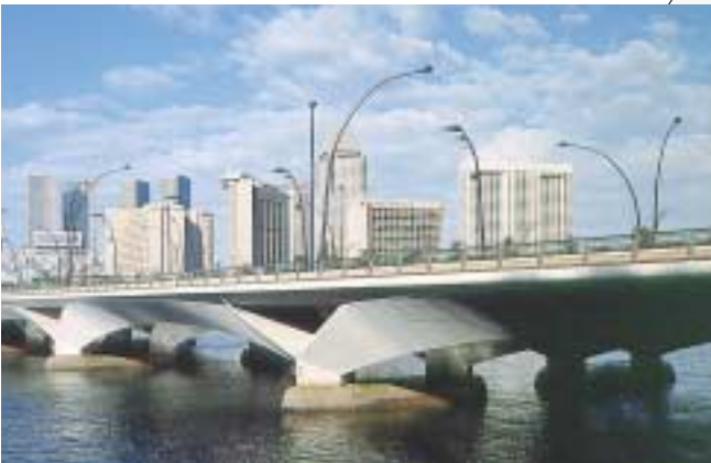
Esplanade Bridge in Singapore
