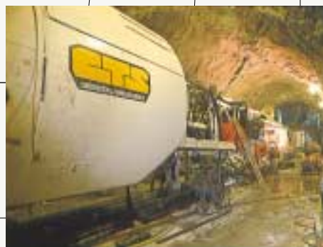
Metro West Drainage Tunnel in U.S.A.
