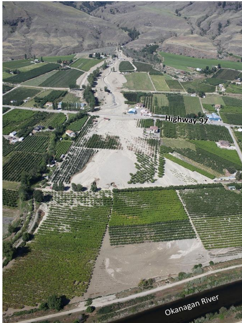
Figure 18: The failure of a very small dam in the uplands triggered a debris flood that emanated from Testalinden Creek canyon (upper centre of photo) and scoured debris load that had accumulated in the channel for years. (Photo credit: Dwayne Tannant CC BY-NC).
