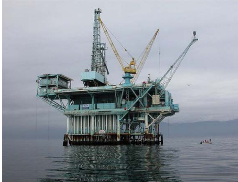
Figure 4.6. Platform A, an example of an integrated topside design (source: http://bayneweb.com/images/blogPics/flkr/oilPlatform.jpg , accessed January 29, 2010).
