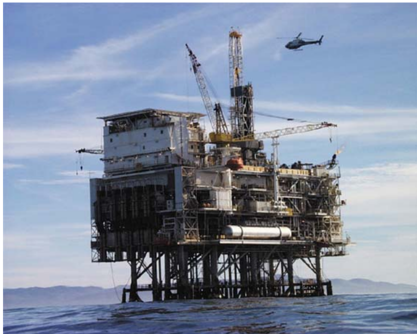
Figure 4.7. Platform Harvest, an example of a hybrid topside design (source: http://www.cosmic.ucar.edu/oceanPI2008/photos/harvest_platform.png , accessed January 28, 2010).
