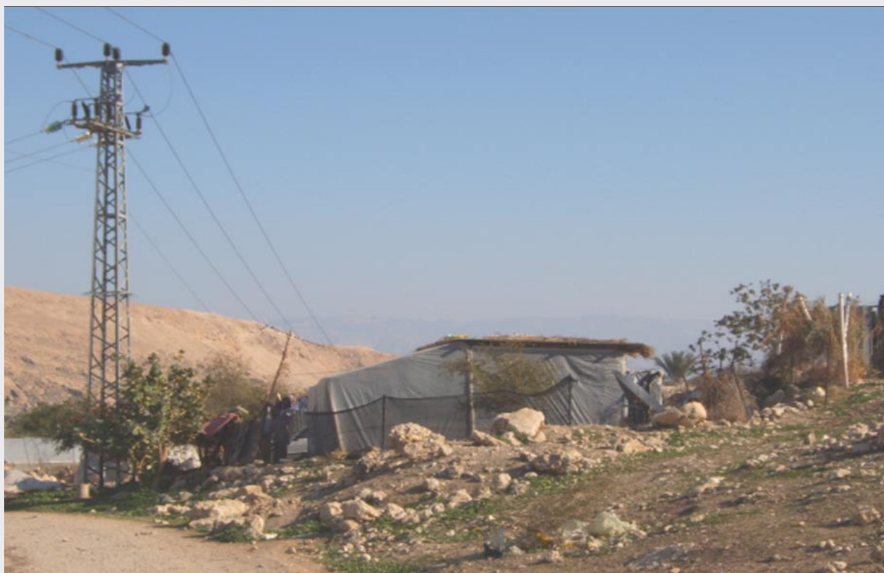
Power lines passing over Al Jiftlik village to provide electricity to nearby Israeli settlements. Photo by OCHA, 2007.
