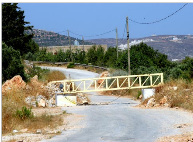
Roadgate blocking access onto Road 60 for Beitin villagers, Ramallah governorate. Photo by J.C.Tordai, 2007
