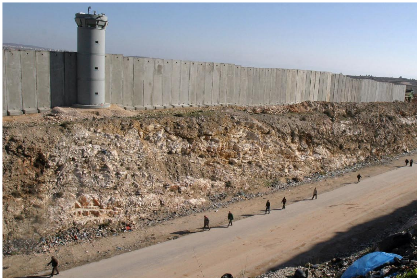
The Barrier along Road 60 from the Palestinian neighbourhood of Ar Ram to Qalandiya checkpoint. Watchtowers and other surveillance measures augment the nine-metre high concrete wall. Much of the Barrier in East Jerusalem is made up of such concrete features. Photo by OCHA/ Steve Sabella, 2005.
