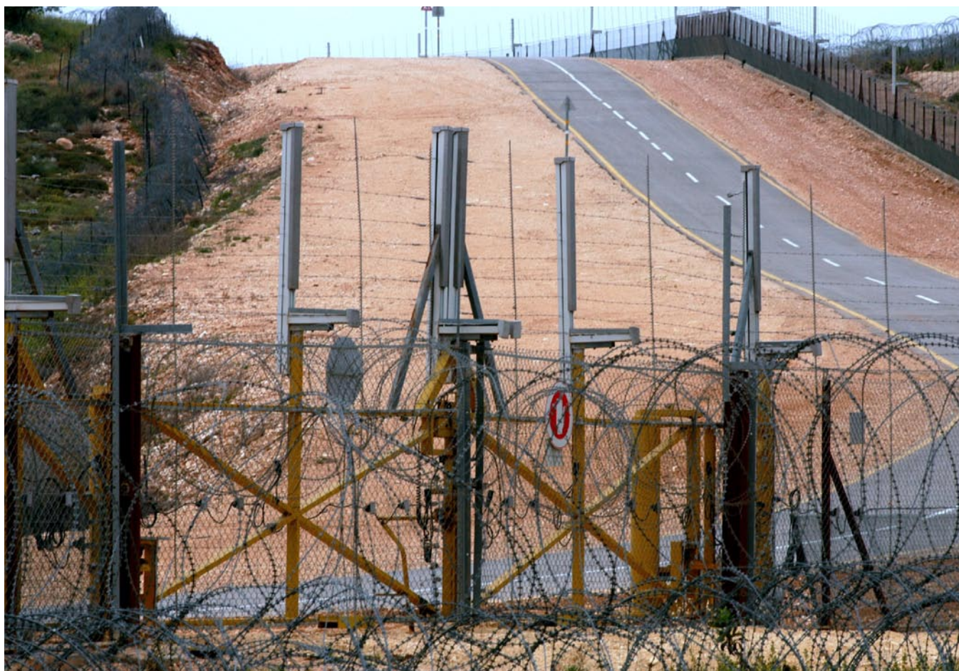
The Barrier near the Palestinian village of Ras 'Atiya (Qalqiliya). The majority of the Barrier is fence-like, made up of a series of electronic fences, patrol roads, ditches and razor wire up to 70 meters wide. It cuts a wide footprint through the West Bank, destroying trees, agricultural land, and irrigation systems. Photo by J.C.Tordai, 2007.
