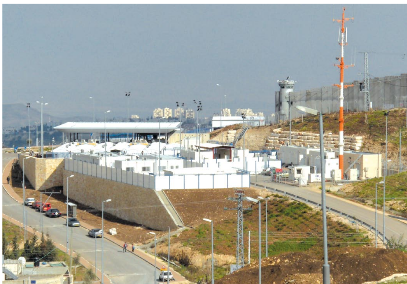
The newly constructed Ras Abu Sbetian checkpoint. This pedestrian only checkpoint is one of only four checkpoints open for West Bank Palestinian ID holders with Israeli issued permits to access East Jerusalem. Photo by OCHA / Nir Kafri, 2007.
