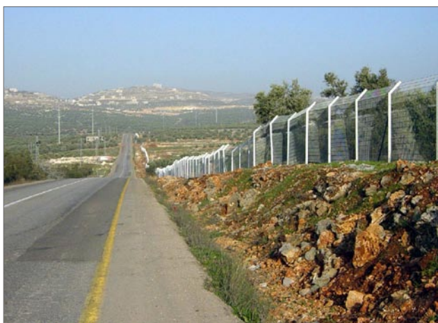
Road barriers along Road 505, Salfit governorate. Photo by OCHA, 2007.
