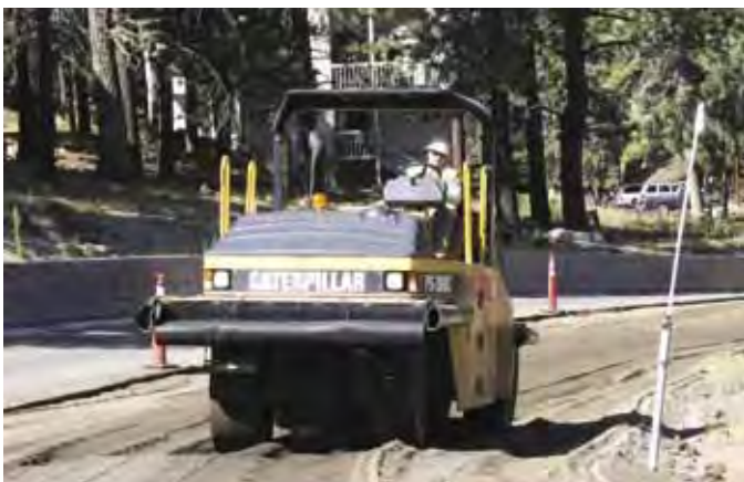
Roller Operator Kelly McQueary flattens the dirt after it's pulverized.
