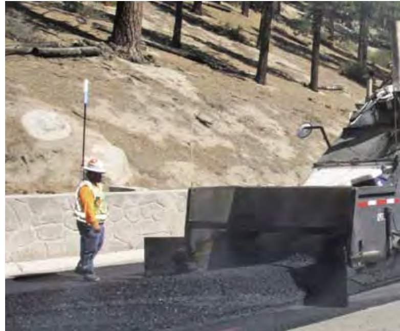
Shuttle Buggy Operator James Brown leads the paving operation down the hill with direction from Foreman Albert Mamac, left.
