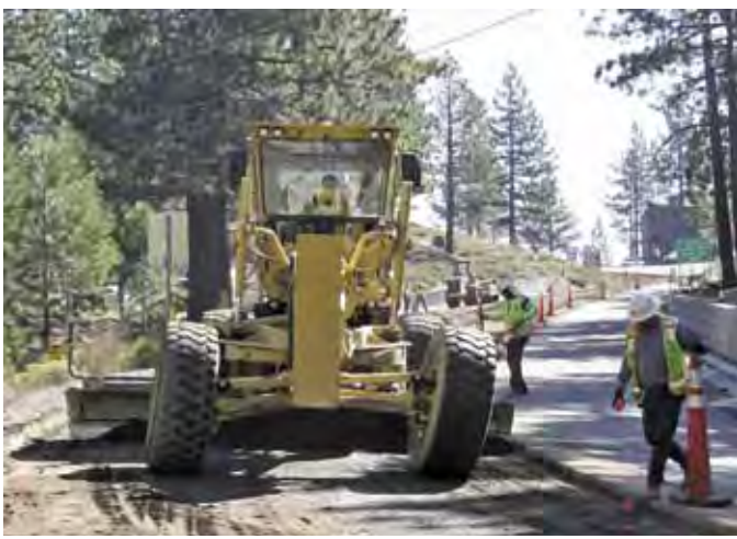
Blade Operator Brad Gillespie makes grade with help from Gradesetter Juan Martinez, right.
