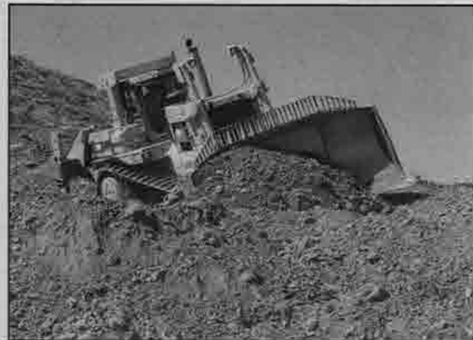
AT WORK: An operator bulldozing material to grade.
