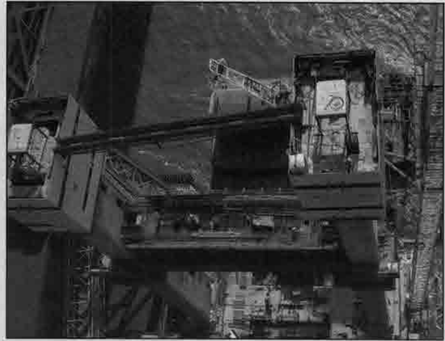
A view of Tower Three from the top of a crane.
