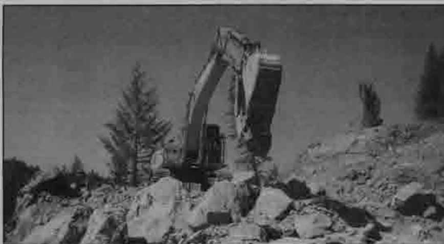
Hugh Shannon operates his excavator.
