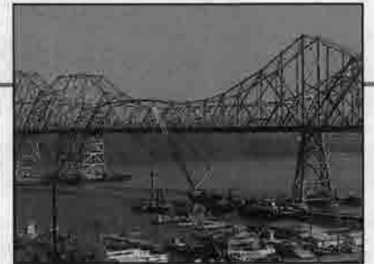
Rebuilding a Giant ..... p. 11-13
