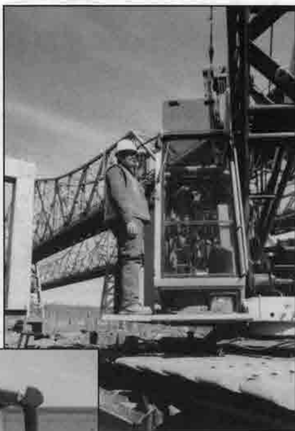
Operators atop a crane at the Carquinez project site.
