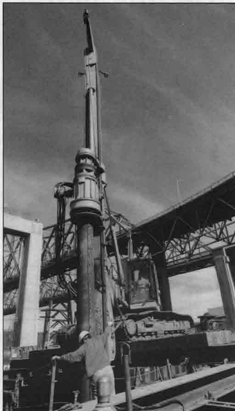
An equipment operator sets pipe at the base of the Carquinez.
