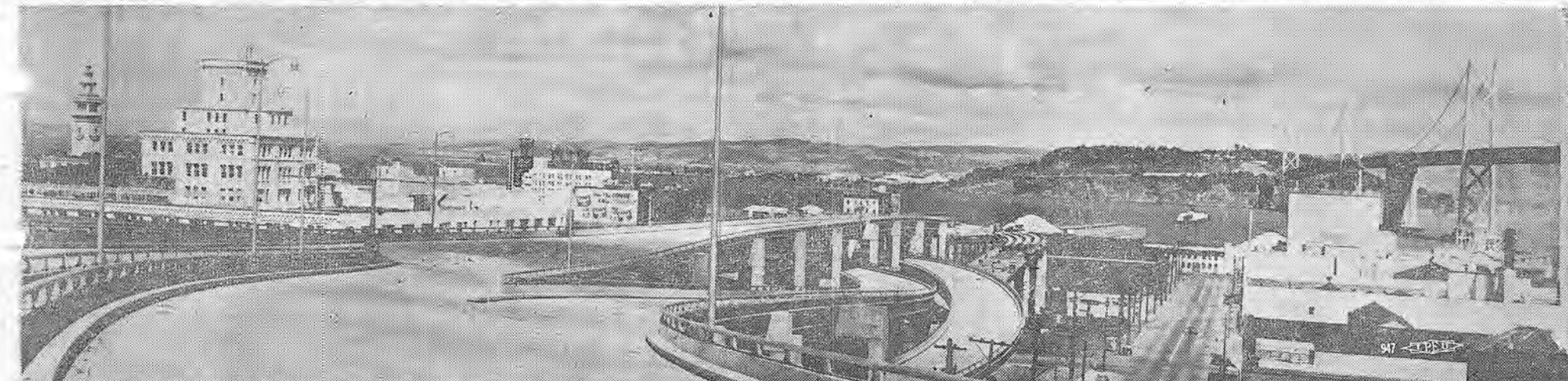
THE VERY OLD AND THE VERY NEW—A massive four-level interchange comparable with the key structure in L.A.'s billion-dollar freeway net is this swooping skyway sculpture where you can get on the mainline for New York, Mexico City, or Vancouver, B.C.—if you read the signs carefully. This construction masterpiece is the heart of San Francisco's freeway network, the newest in transportation, contrasting sharply with the old, picturesque, and restful mode presented by the ferry crossing the Bay. Behind us lies the giant Bayshore skyway, to the right is the Bay Bridge, and dead ahead Embarcadero Freeway, which will take you along the waterfront in front of Ferry Building, at left. Picture was taken day before some of these ramps were opened to carry downtown traffic to Bayshore. (Staff photo)
