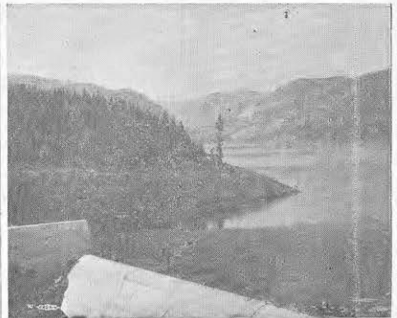
This view of the Cherry Valley Dam over the spillway was taken shortly after Lake Loyd formed by the dam began to fill. To the left of the picture is the north abutment of the dam while the spillway is to the right. The last visit to the dam showed the lake now about one-third full.
