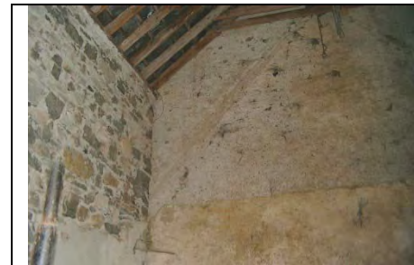
Outbuildings – internal view indicating original roof line
