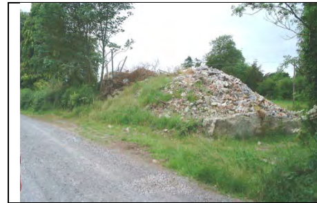
Demolished House, Ballingar Road
