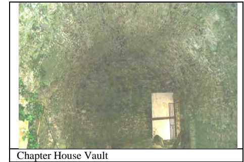
Chapter House Vault
