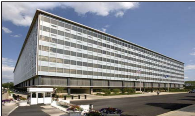
Figure 2: The Coast Guard’s Headquarters Building
