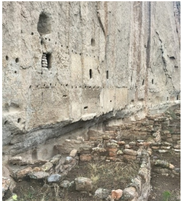
Figure 16. Holes cut into cliff faces at sites like this one in Bandelier National Monument, NM, confirm that some holes in bedrock were used as pole sockets (Photo by Chris Reed)
