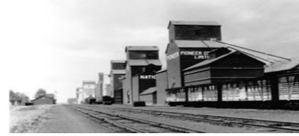
5) Elevator Row 1909 - 2003 49th Ave. & 48th St. to 52nd St.
