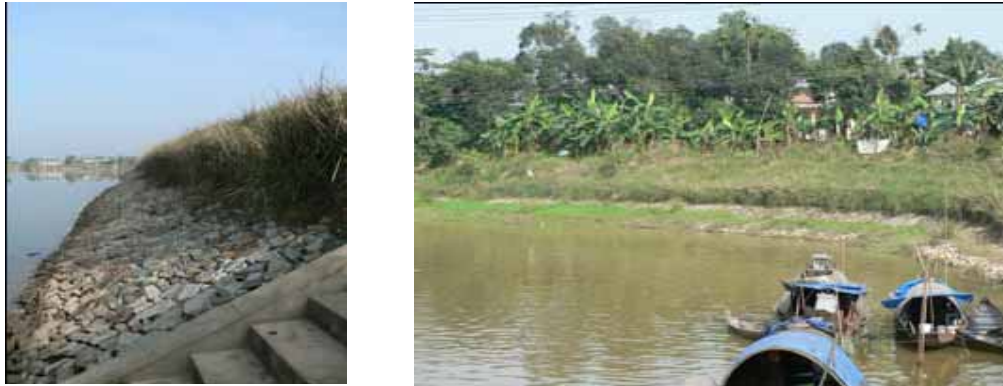
Photo 10: Left: Vetiver and rock riprap (upper) and concrete frame (lower) protect an embankment; right: a bend on Perfume Riverbank in Hue
