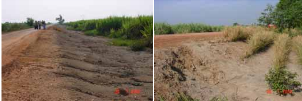
Photo 21: Before and after Vetiver installation in extreme acid sulphate soil on an embankment in Tien Giang province, Vietnam
