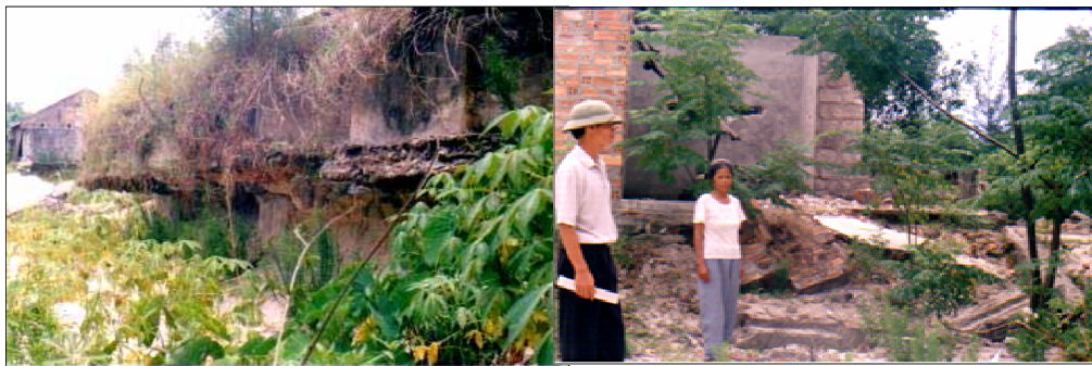
Photo 2: Sand flow in Le Thuy (Quang Binh) in 1999. Left: the foundation of a pumping station; right: this woman's three-room brick house
