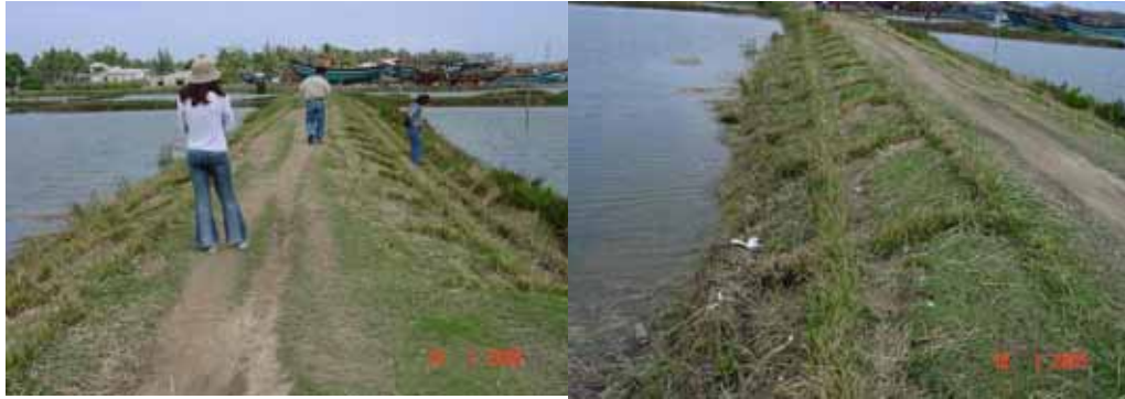
Photo 24: Vetiver, installed in a cross-hatched pattern, protects shrimp pond dikes in Quang Ngai
