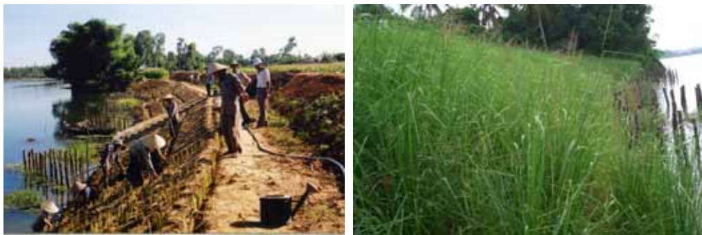
Photo 14: Left: Community members plant Vetiver; right: November 2005: bank remains intact following the flood season
