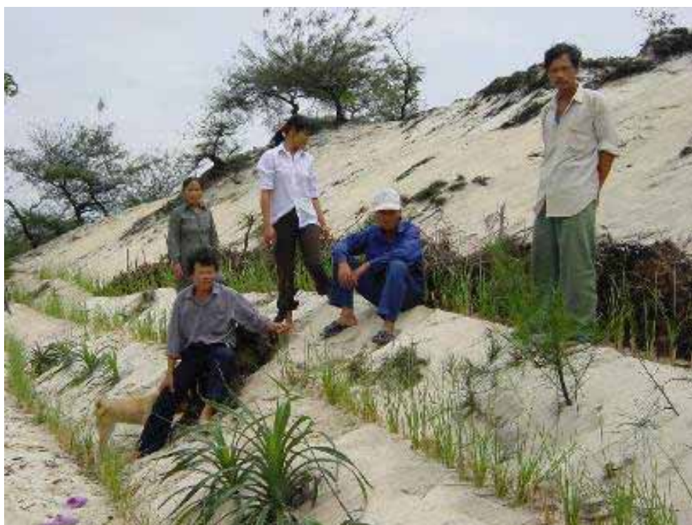
Photo 15: Early April 2002 – Vetiver one month after planting. Note: Mulch was put above the top row.
