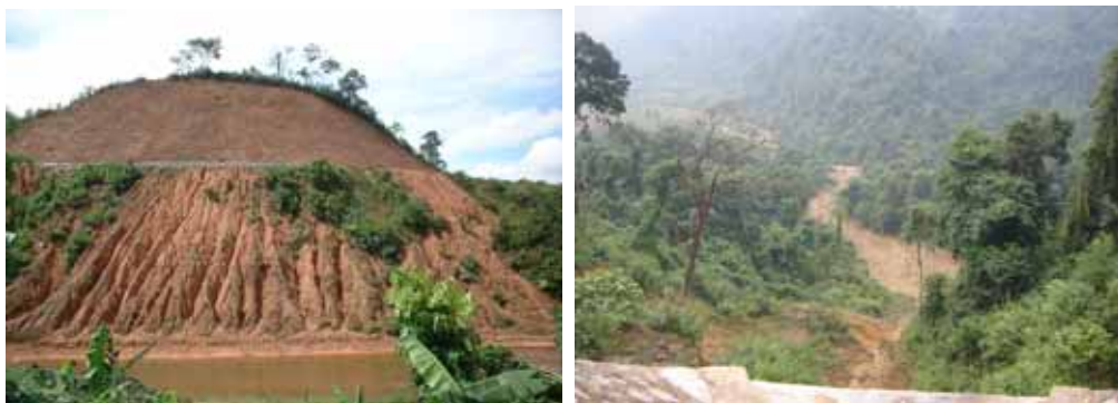
Photo 20: Left: Improper rock/soil waste disposal moves far downstream; right: impacting a village in A Luoi district, Thua Tien Hue province
