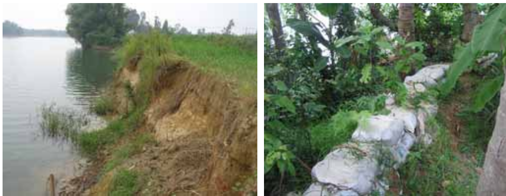
Photo 13: Left: severely eroded bank of the Tra Khuc River, at Binh Thoi Commune; right: primitive sand bag protection
