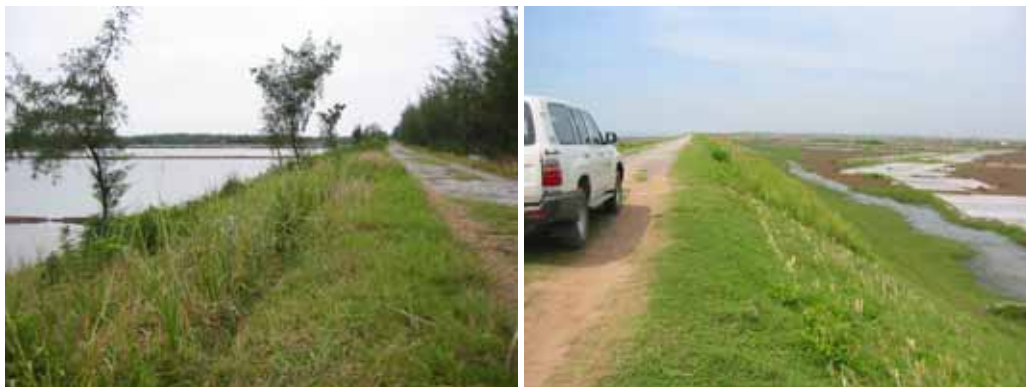
Photo 18: In North Vietnam; left: Vetiver planted on outer side of a newly built sea dike in Nam Dinh province; right: on the inner side of the dike, planted by the local Dike Department
