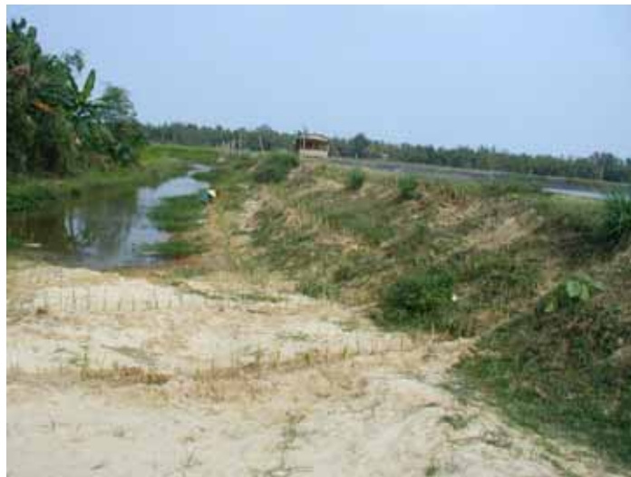
Photo 23: Vetiver protects a shrimp pond near a natural gully that drains water into a river (Da Nang province); this model was established as part of the first Vetiver project financed by the Royal Netherlands Embassy in Vietnam
