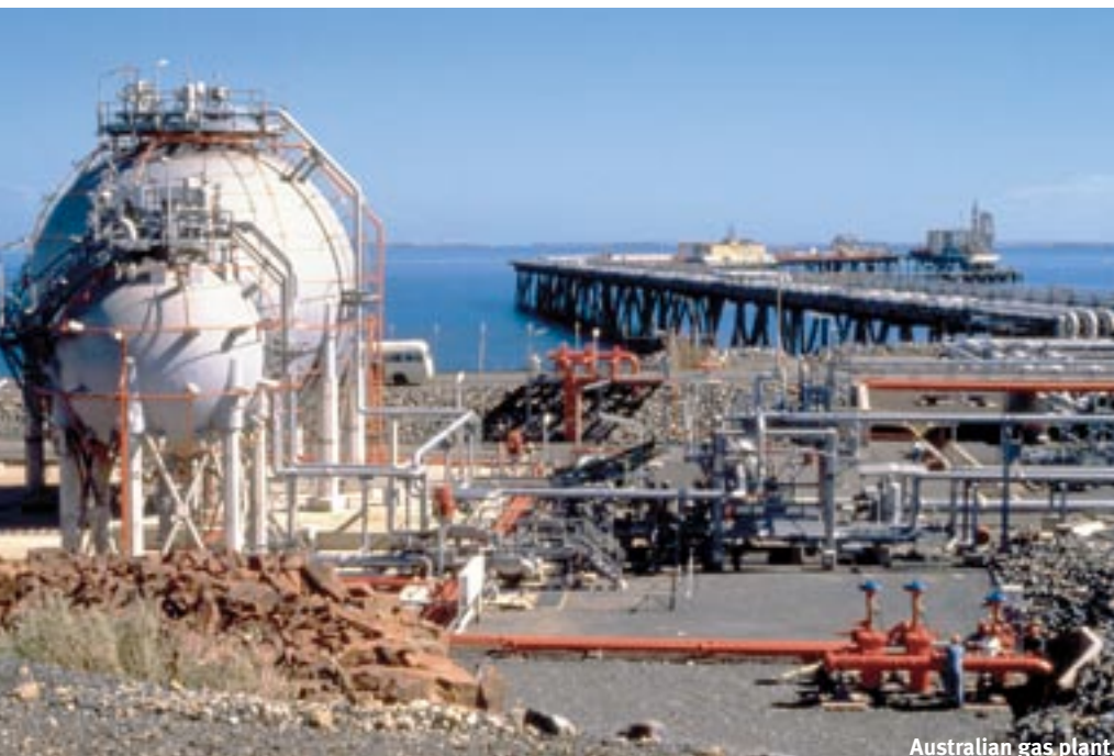
Australian gas plant.
