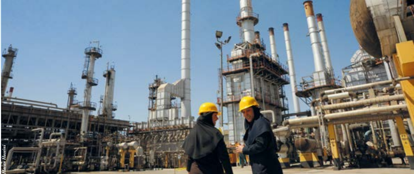
Refinery in Tehran.
