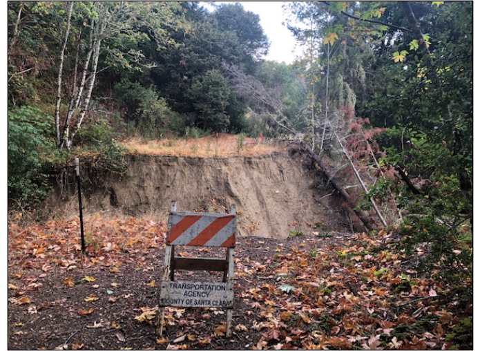
B) Project site with view of proposed landslide repair
