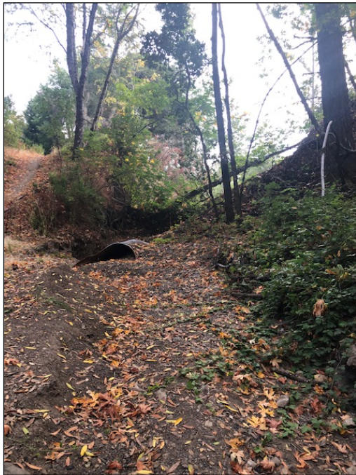
C) Project site with view of proposed culvert repair
