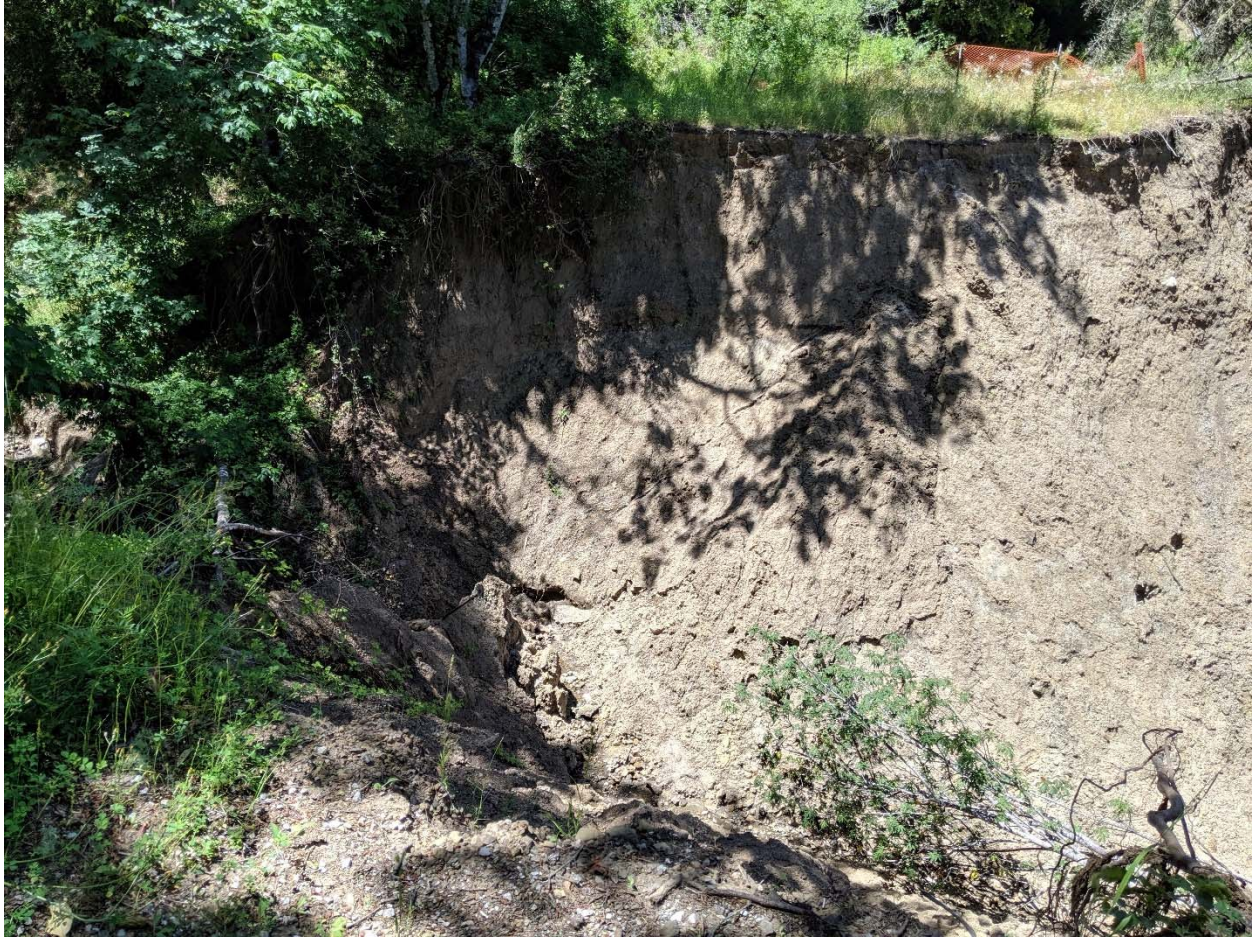
Photo 4. Delineated other Waters at Data Point P01, showing incised, failed slope in eastern portion of study area corridor.
