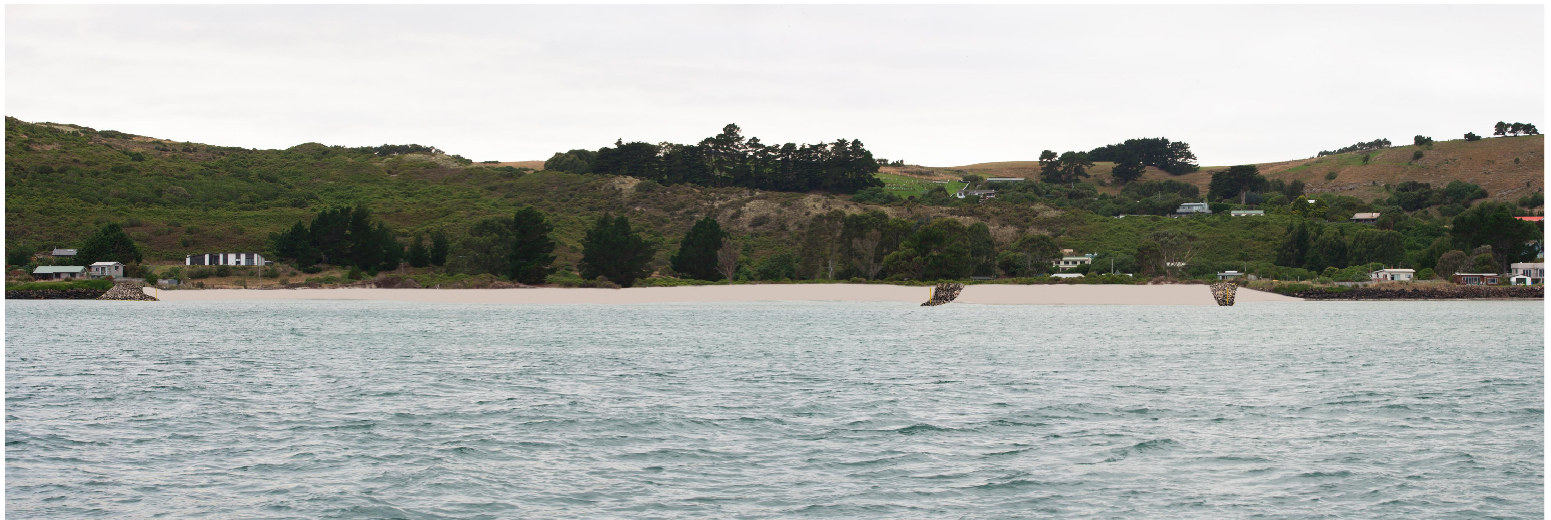
Channel View - (Low tide) with groynes and sand.
