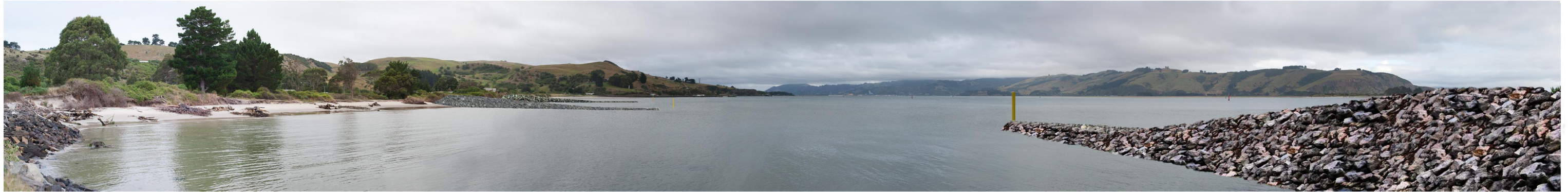
View B - (Low tide) with groynes.
