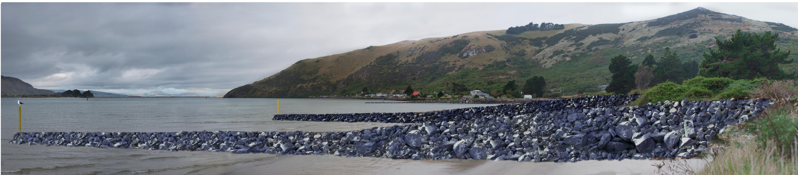
View A (Low tide) with groynes.
