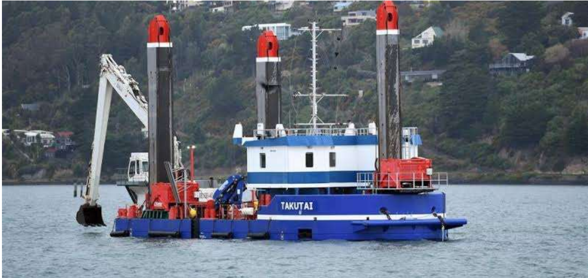
Figure 3: The dredger Takutai. Note that she will be fitted with a suction head, not an excavator bucket, for sand recovery.
