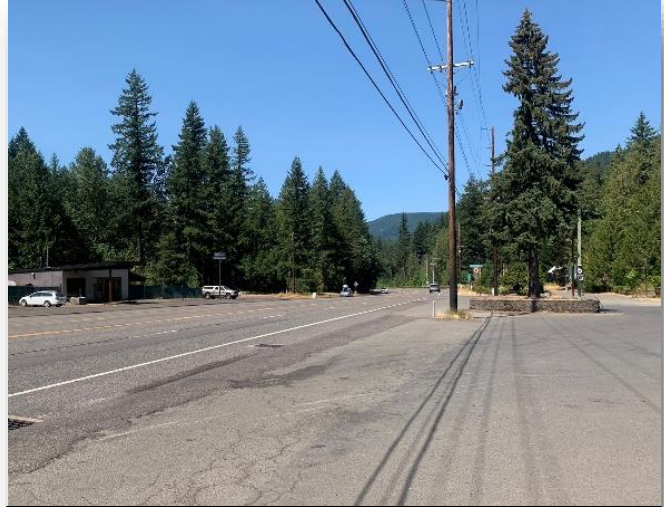
The absence of curbs within the study area provides a lack of access definition and allow for relative high-speed turning maneuvers into adjacent parcels from U.S. 26.
