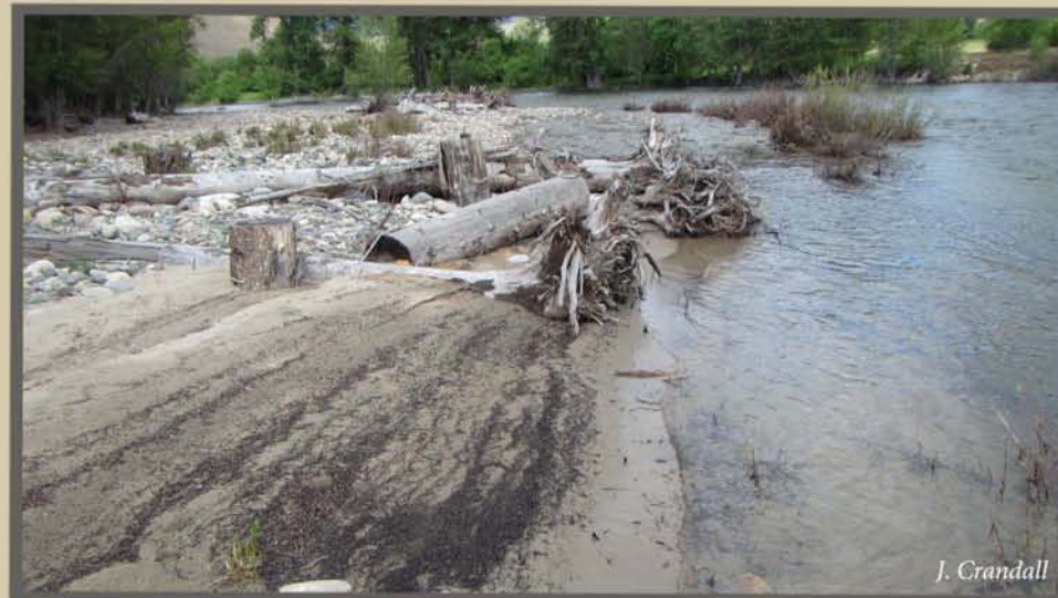
Engineered wood structures, like this example at the Whitefish Island Project in the Methow River, can promote sediment deposition that helps create attractive habitat for ammocoetes.
