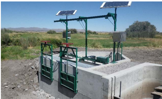
This screen was designed to protect warner sucker and redband trout.
