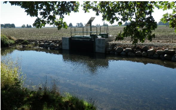
The new belt screen protects fish throughout the irrigation season.
