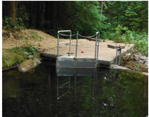
The stream flows perpendicular to the screen reducing the likelihood of fish impacting the screen.
