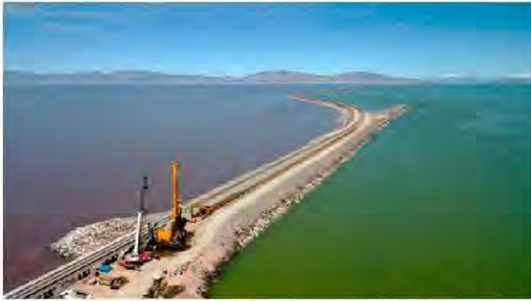
Union Pacific's rock-fill railroad causeway stretches 20 miles across the Great Salt Lake, the largest salt water lake in the Western Hemisphere.
