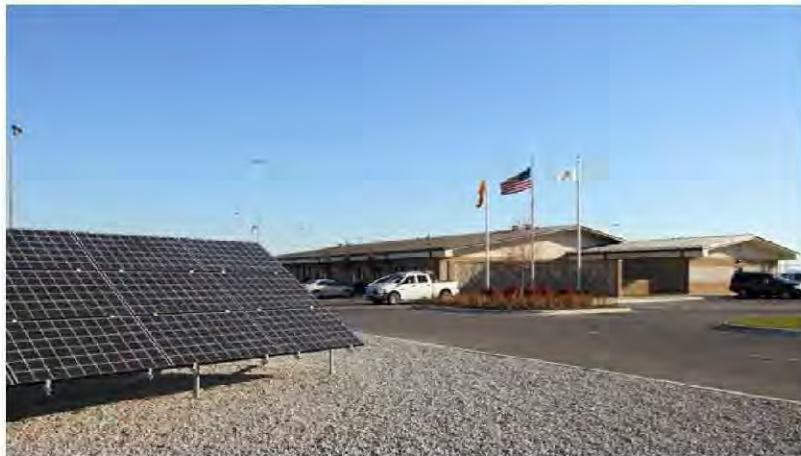
Solar grids at the Joliet Intermodal Terminal near Chicago.
