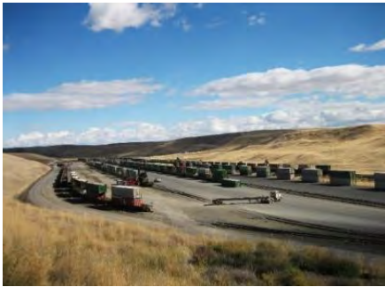
Figure 14. The Columbia Ridge railyard has over 26,000 feet of existing track.
