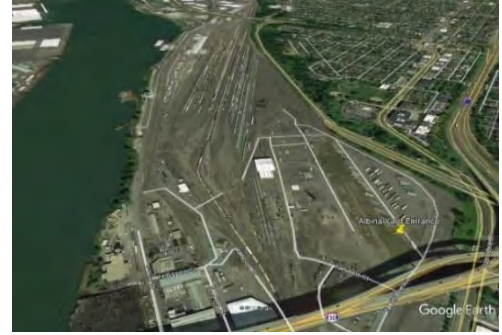
Figure 13. The Portland Albina railyard will have 11,600 linear feet of Metro dedicated track.
