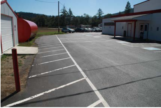
Parking lot "No Parking" zones and pedestrian walkway/crosswalk striping use the same pattern.
