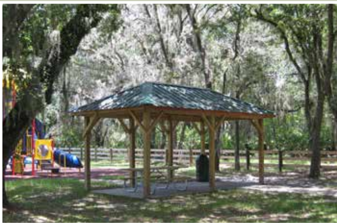
Typical park standard pavilion
