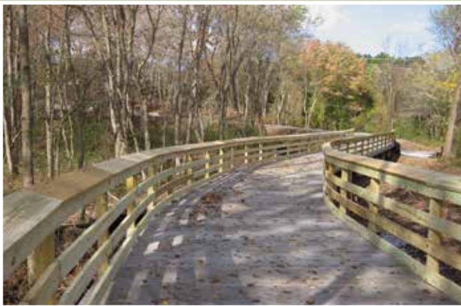
Concrete boardwalk - photo courtesy of Permatrack
