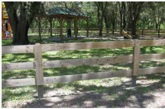
Three rail wooden fence
