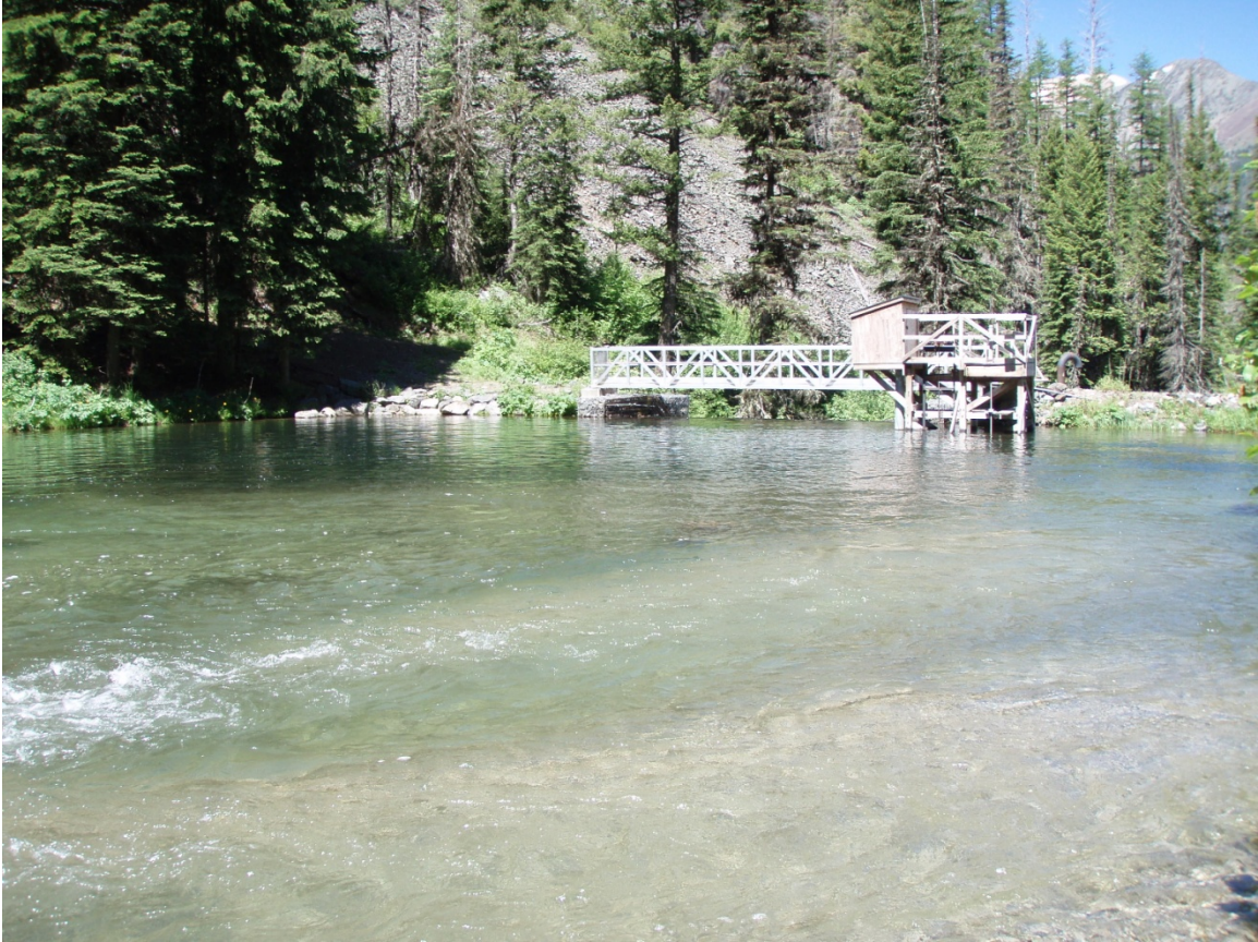
Figure 7: Forebay taken from the SW corner facing NE.
