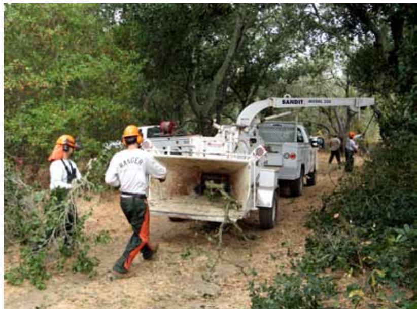
Constructing an ingress/egress zone
