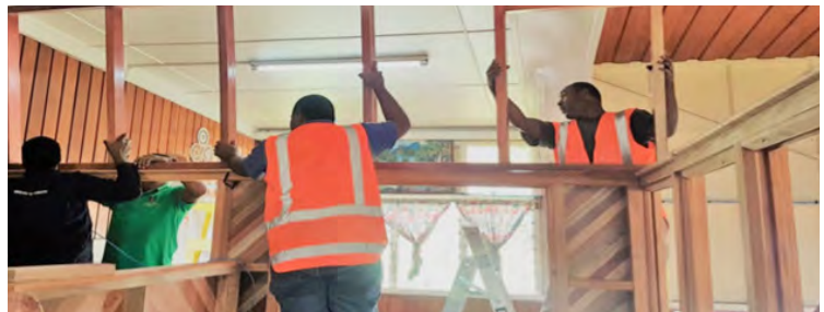
Figure 16: Upgrading of the office reception area
