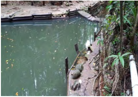
Figure 7: Block laying works at the 2nd pool
