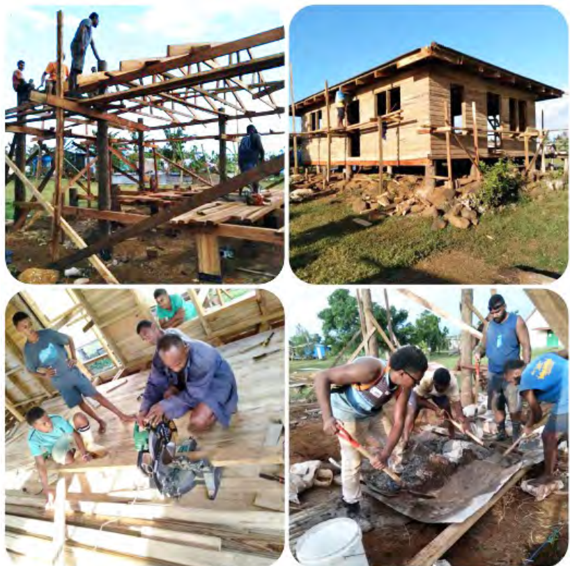
Figure 20: House construction in communities
