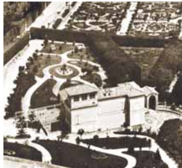
Fig. 233. Aerial view of the Casina Pio IV before the new extension was built.
