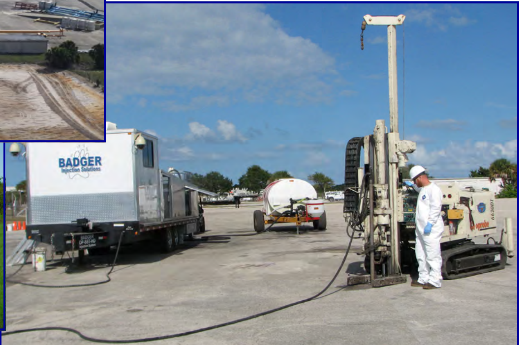
Bottom right: EZVI injection in Hangar K solvent source area (approx 2011)
