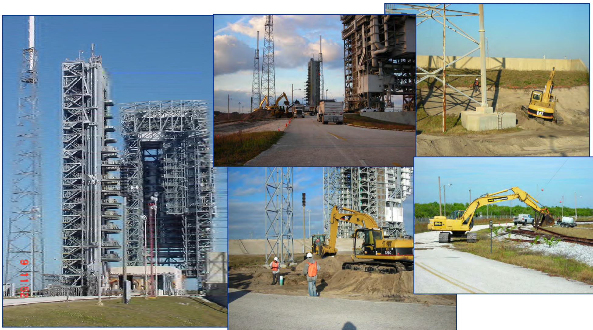
Above left shows launch structure at time of deactivation (2005). Photos at right are of soil removal conducted during deactivation process (2006-2007). Currently, photography at the site is restricted due to the secure nature of the launch complex.
