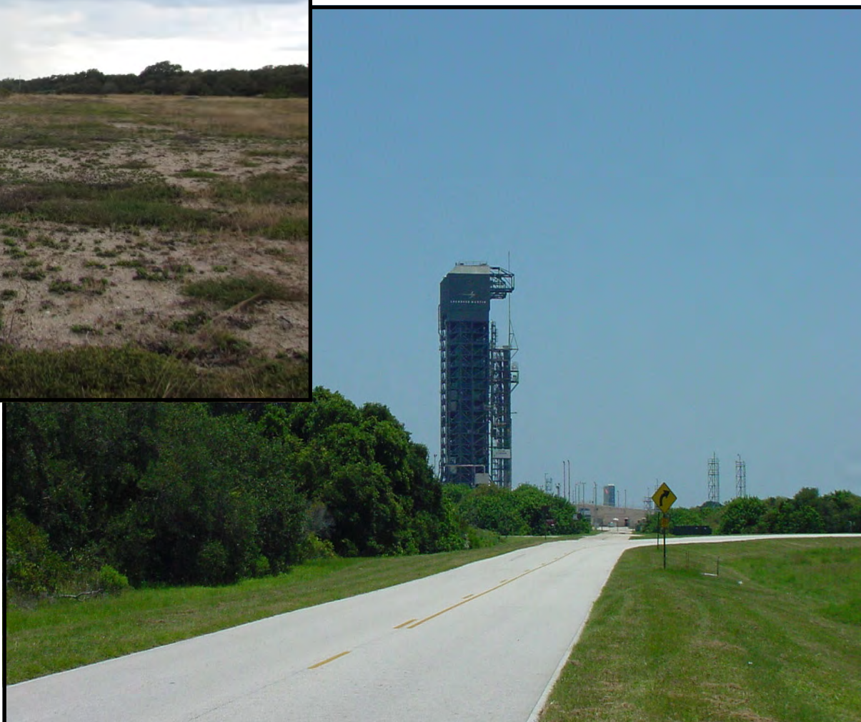
At left: Photo shows conditions at SLC-36B prior to initiation of Blue Origin construction activities. Pad was demolished shortly after deactivation in 2005
