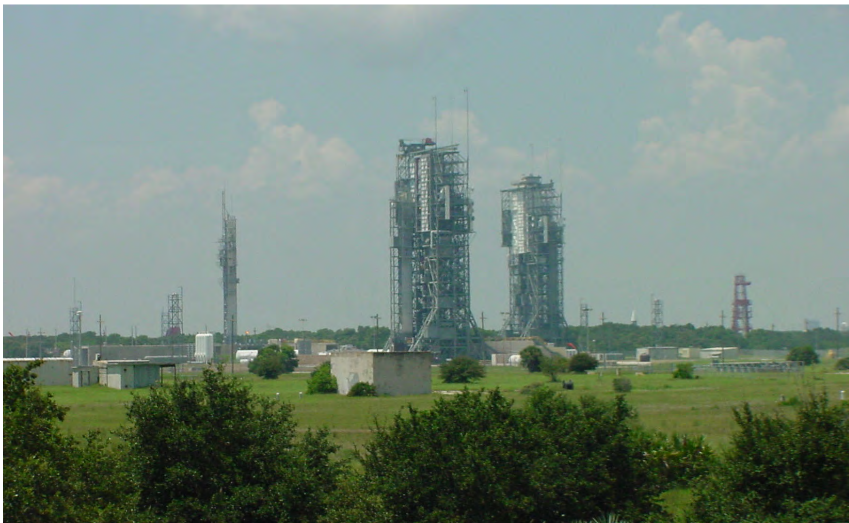
This photo shows an overview of the former launch towers and support facilities at SLC-17. The launch towers were demolished in 2018. This photo was taken from SLC-31/32 facing southwest.
