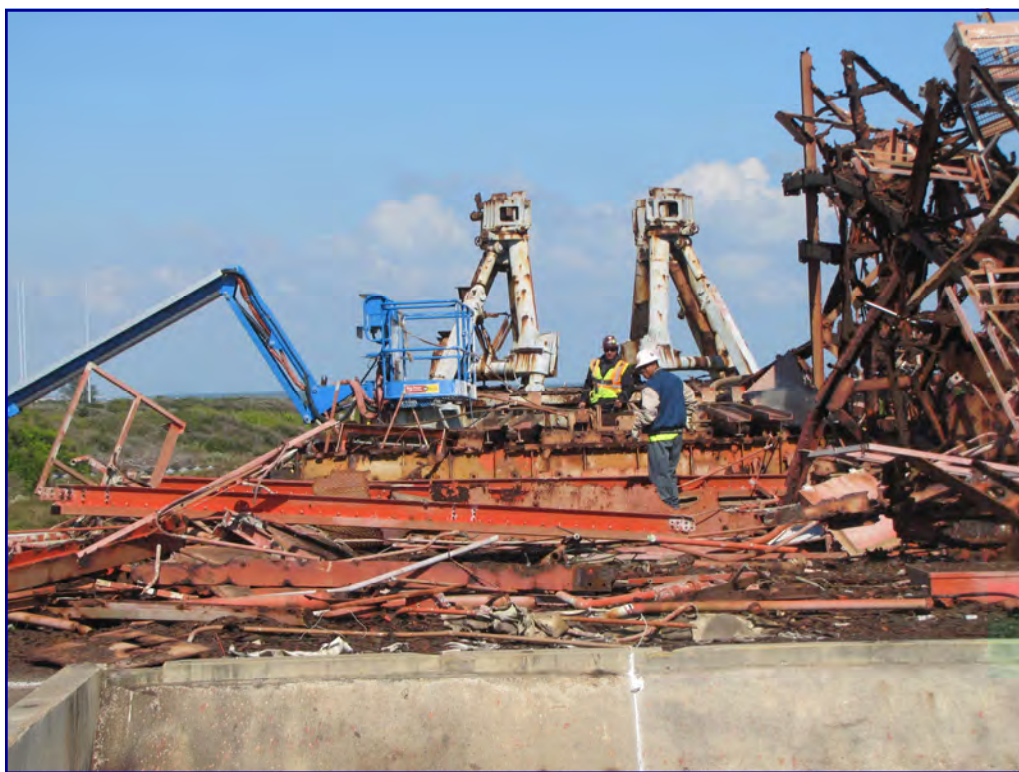
Left: Remaining painted launch structure (on top of launch stand) during demolition and removal (Nov 2012). Below: Same part of launch stand following removal of the painted structures (Dec 2012).
