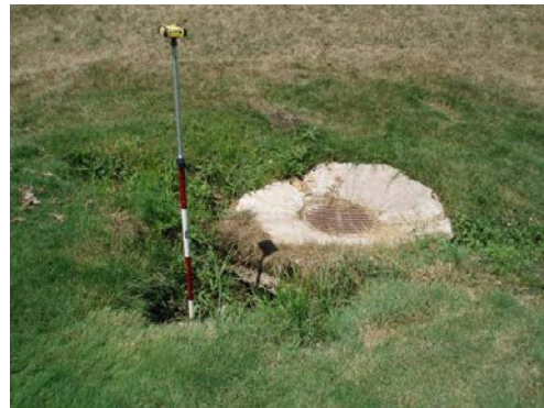
Pipe inlet from east end of golf course parking lot is in poor condition
