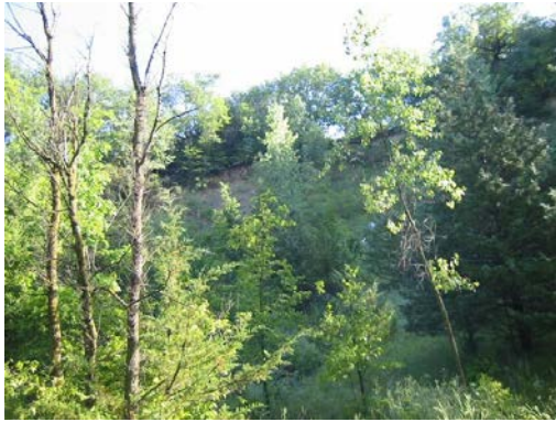
Large slope failure has revegetated the lower bank
