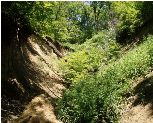
30 foot deep slope failure area
