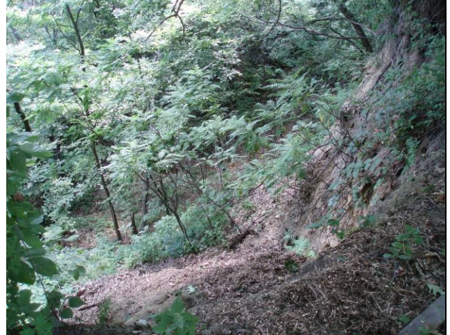
Yard waste dumping onto failed slope
