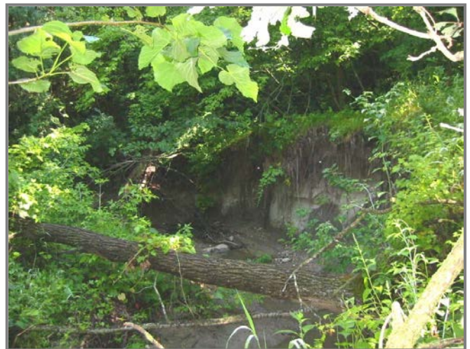
Figure 38 Severe bank erosion is found in the 400-foot reach of Bluff Creek at Site 20. Flow causes and determines the degree of streambank erosion in Bluff Creek.
