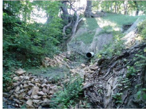
New pipe outlet from golf course
