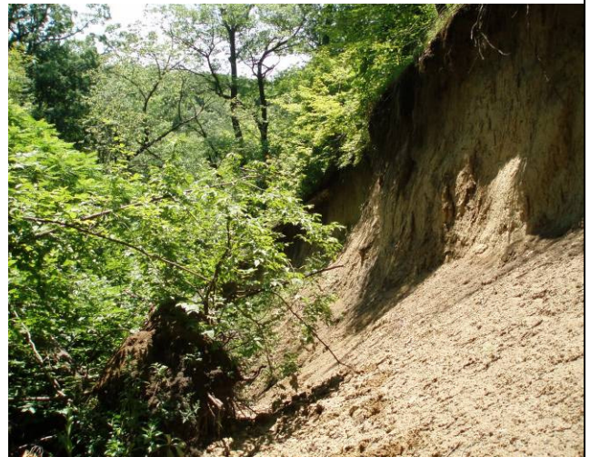
Typical failed sidewall
