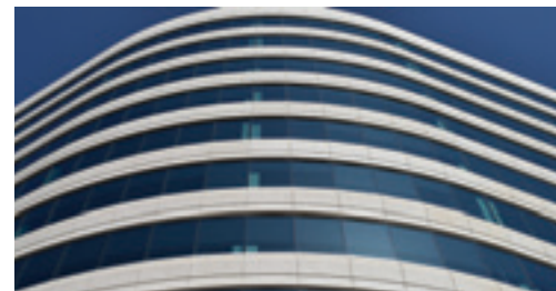
Precast elements add style and efficiency to the CoBank building in Greenwood Village, Colorado. Photo: Rocky Mountain Prestress.
