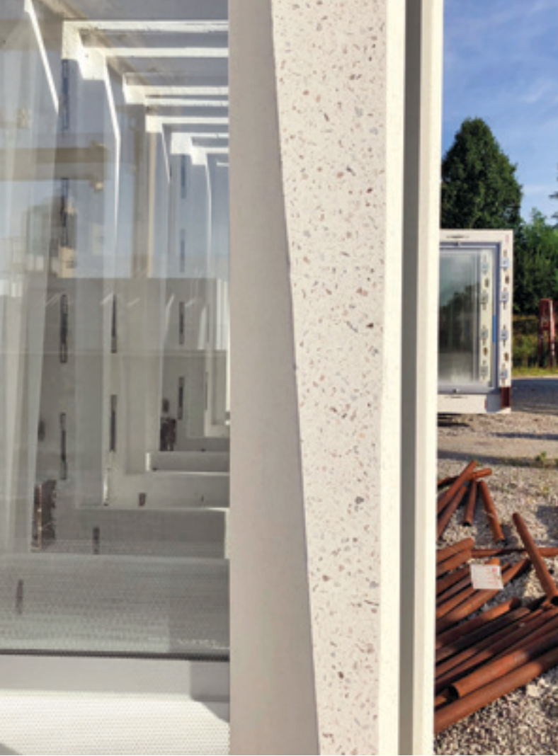
At the former Domino Sugar factory site, deep white precast concrete panels frame the windows and emulate the structure of sugar crystals. Units are ready to be shipped to the project in Brooklyn, N.Y. Photo: Gate Precast.
