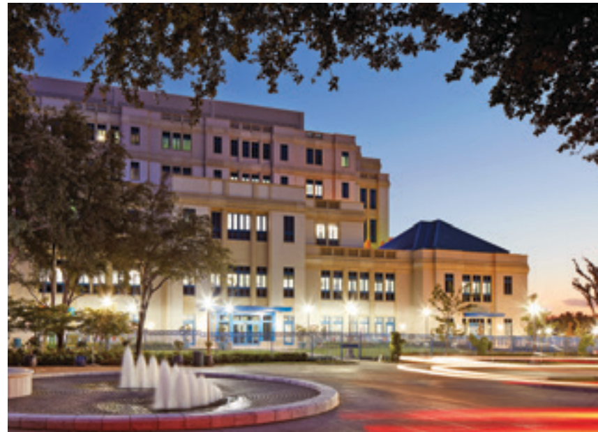
Seen here at dusk, the new South Tower bookends the garden forecourt and main entry drive to the Medical Center.
