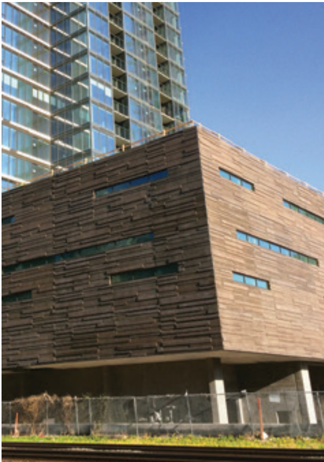
The new Marriott Hotel and apartment tower in downtown Calgary, AB, Canada, includes a five-story parking structure and 10,000-ft 2 conference center at its base clad with precast concrete panels featuring a custom-finished formliner that creates a stepped-ribbed finish with smooth-, fine-, and coarse-grain finishes on individual ribs. Photo: U.S. Formliner.
