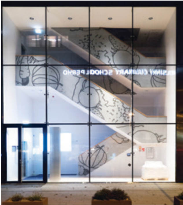
The Helsinki Culinary School used the Graphic Concrete technique inside the building to depict fruits and vegetables used in the school. Photo: AltusGroup.
