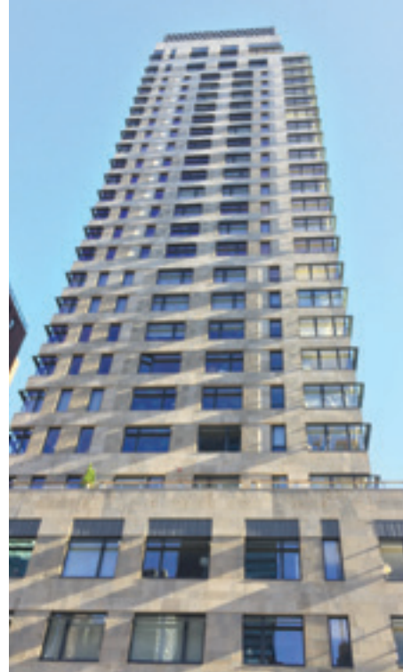
This midtown development located at 301 East 50th Street is a thoughtful balance between well-proportioned windows, precast concrete with limestone walls, and sun shading create a comfortable, yet expansive and panoramic, view of the city.
