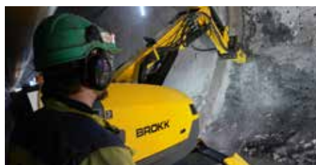
Remote controlled units physically distance employees from harmful silica dust, as well as the strong vibrations of handheld equipment such as breakers, rivet busters and chipping guns.
