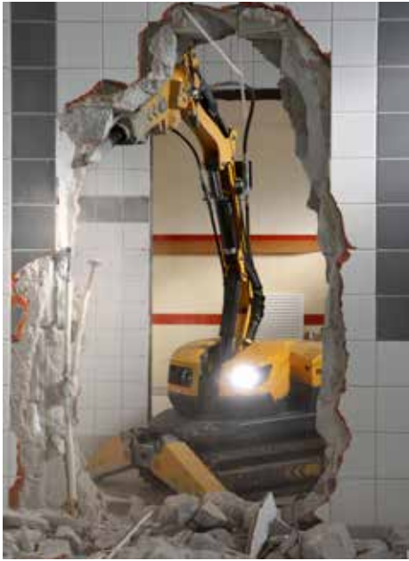
Thanks to advanced technology and an industry leading power to weight ratio, compact demolition robots can access some of the most restrictive jobsites.
