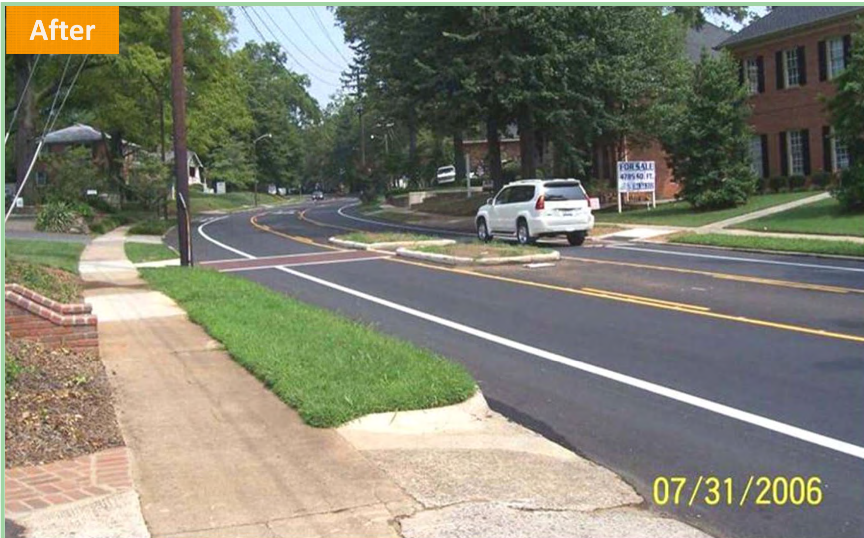
Reclaiming road space creates room for ped islands
