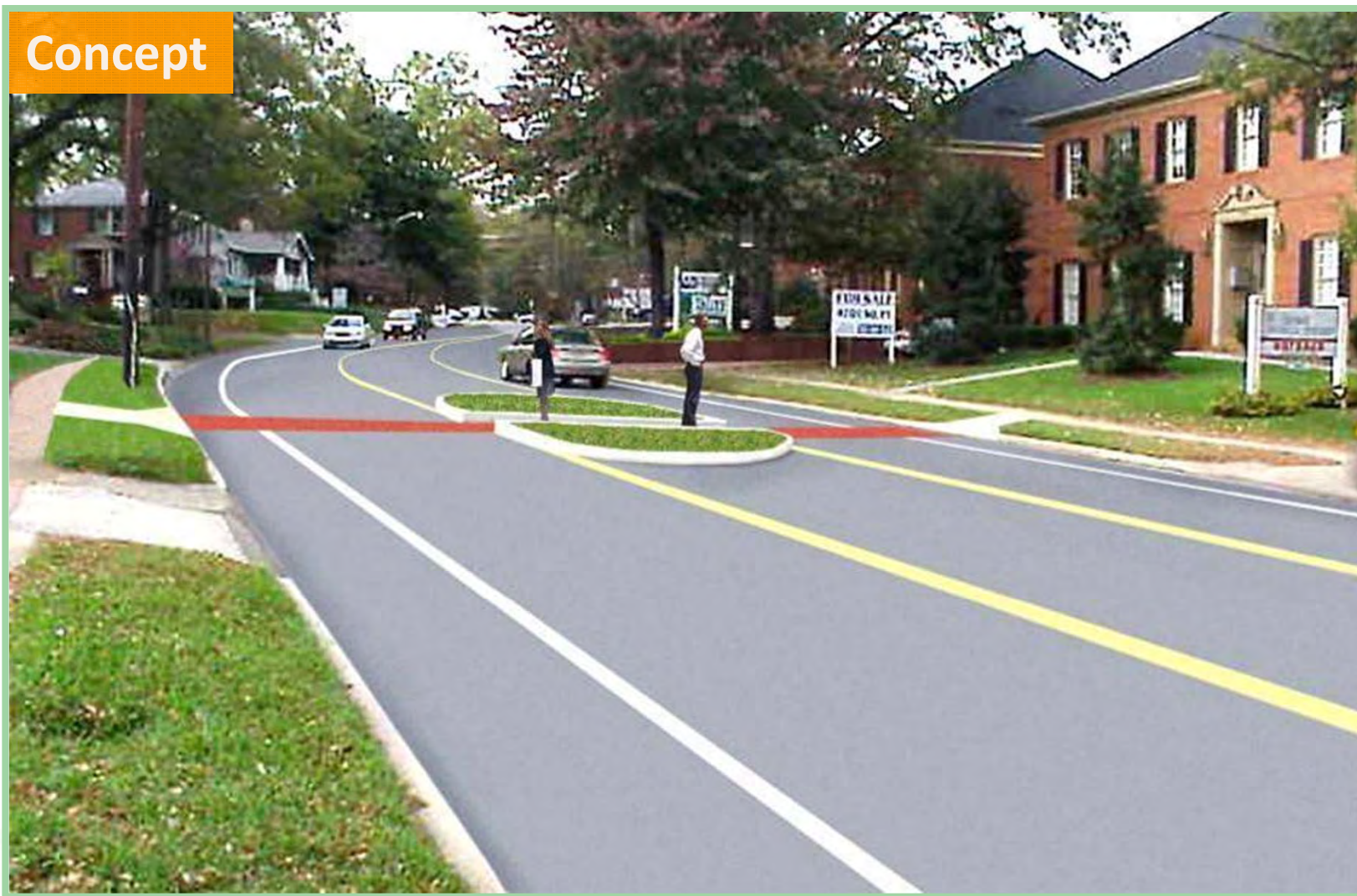
Reclaiming road space creates room for ped islands
